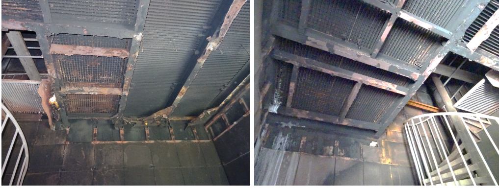
Figure 17: Floor steel beams above the first floor near spiral staircase, “ZONE 3”.
