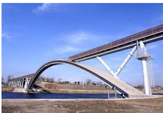
Obr. 22 Most míru – Seonyu Bridge (21)
