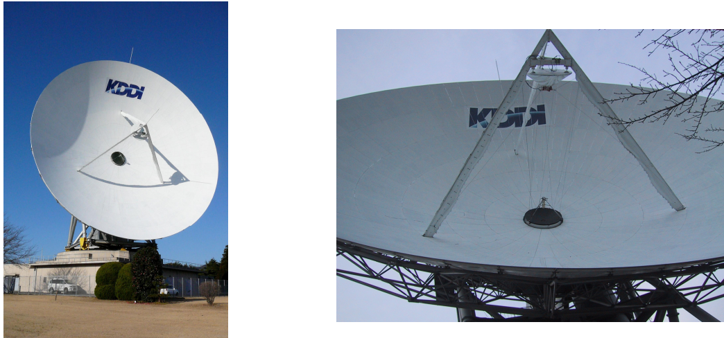
Fig. 10 - KDDI antenna equipped with 2m, 70cm and 23cm feeds.
