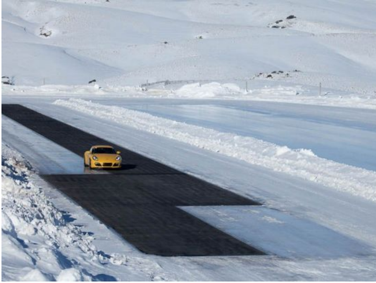
Figure 4.4: An example of split \mu road on a testing site; picture taken from [16]
