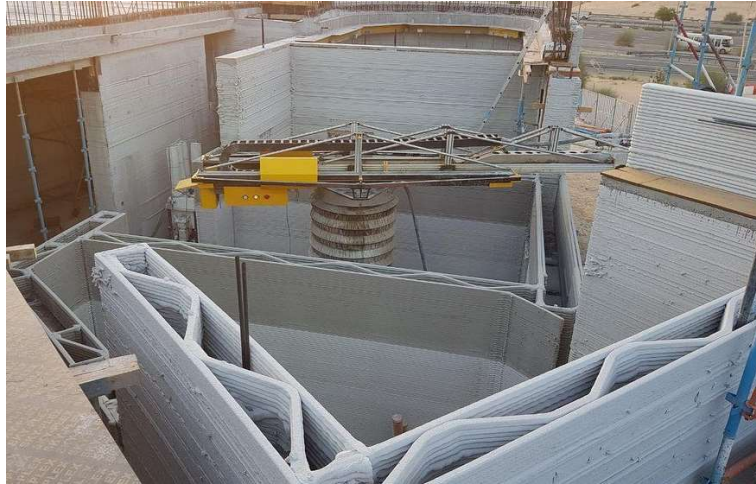
Figure 2-28: 3D-printed in-situ concrete wall by Apis Cor [Api19]
