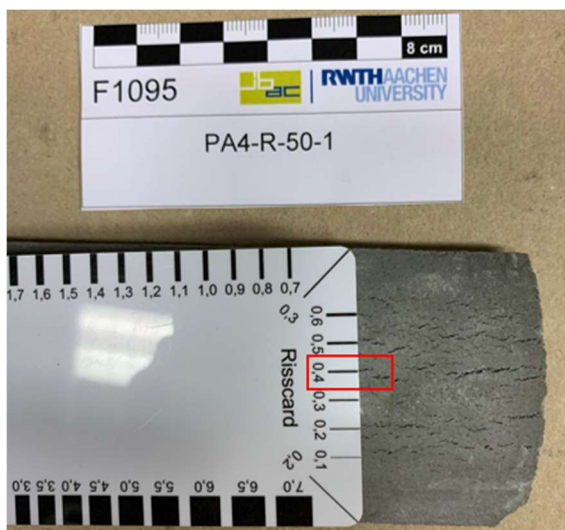
Figure 5-3: Measurement of crack width
