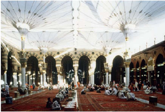
Figure 3-1: Prophet's Mosque in Madinah, Saudi Arabia: convertible umbrellas [Lew17c]
