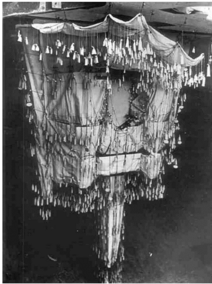
Figure 3-4: Gaudí's hanging model [Mah03]
