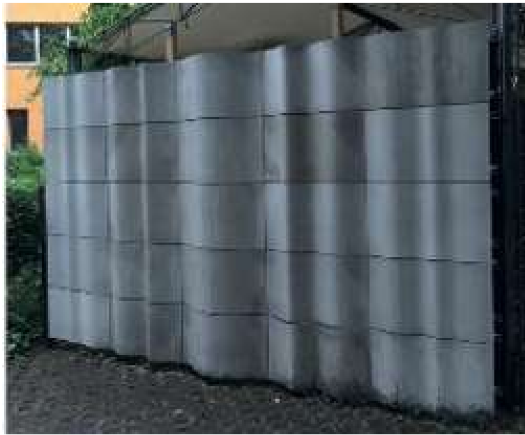
Figure 2-21: Prototype wall made from 25 folded TRC elements [Pid16]
