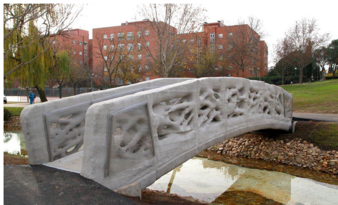
obr.114 3D Printed Bridge (2016), Madrid - Španielsko, IAAC Institute for Advanced Architecture of Catalonia/ D-Shape [17.9]
