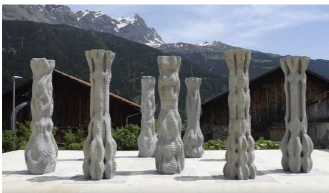
Obr. 7 3D Printed Concrete Columns (2019), Švajčiarsko, ETH Zurich/NCCR DFAB [7]
