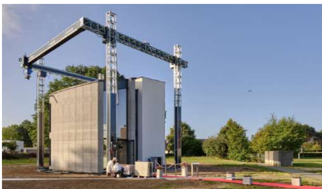
Obr. 3 Kamp C 3D House (2020), Westerlo - Belgicko, Kamp C, COBOD [3]
