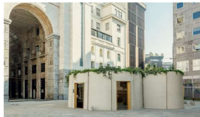
Obr. 4 3D Housing 05 (2018), Mlano - Taliansko, CLS Architetti, Arup, CyBe [4]
