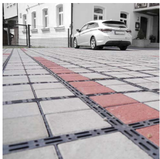
Ecoraster Bloxx/ infiltration pavement [24]
