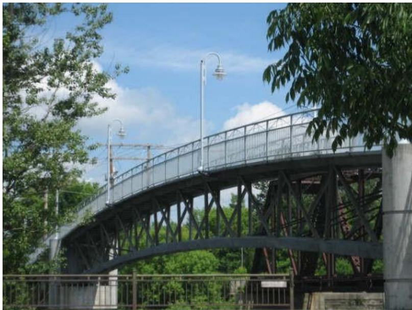
Obr. 28 Sherbrook Footbridge, Kanada [36]
