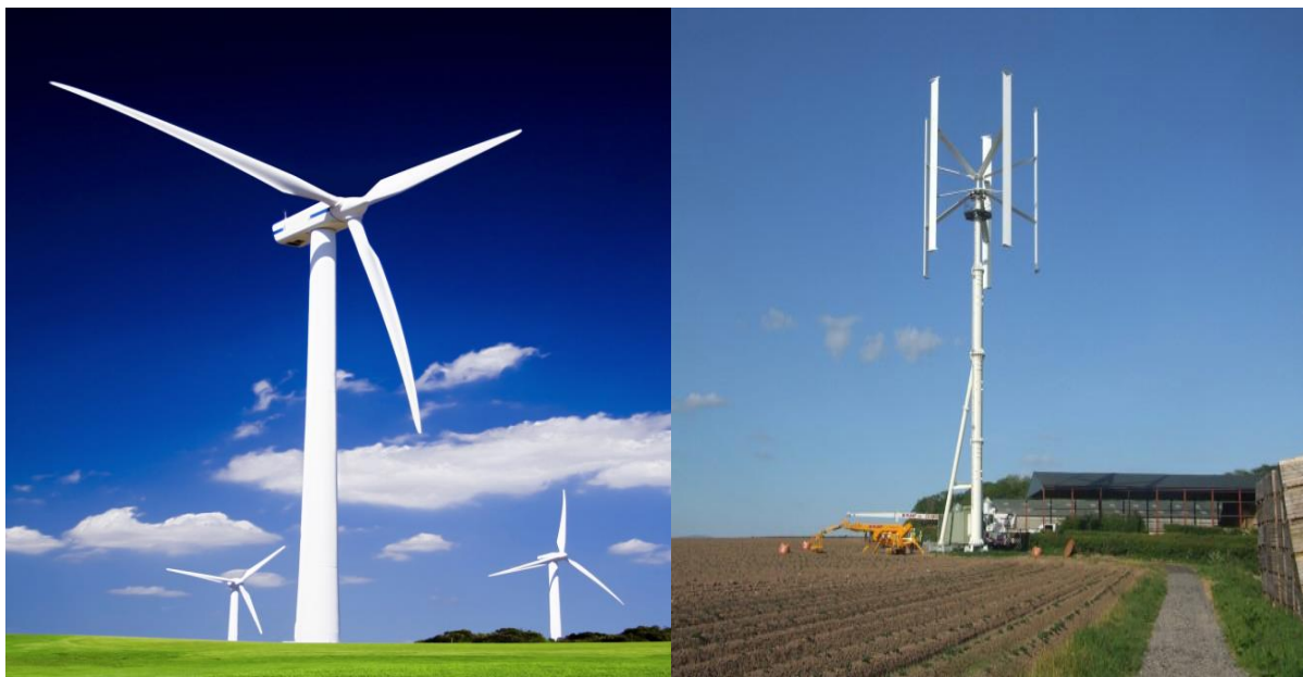
a.Horizontal axis wind turbine
