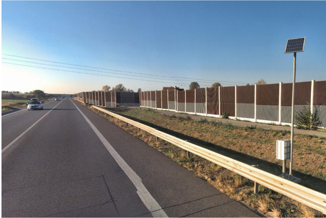
Figure 13: An example of SATC (Marksman 680) powered from solar panel (18)
