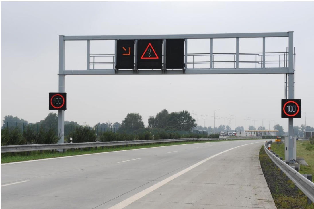
Figure 23: Example of highway line traffic management in operation
