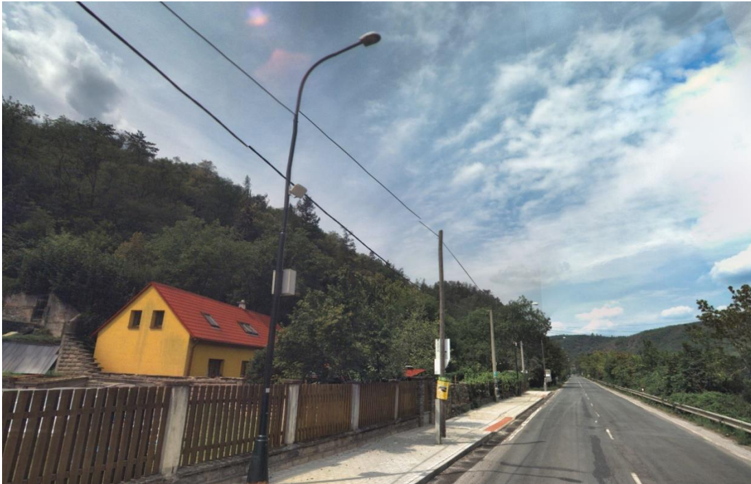
Figure 14: An example of SATC (Wavetronix) powered from public lightning (18)
