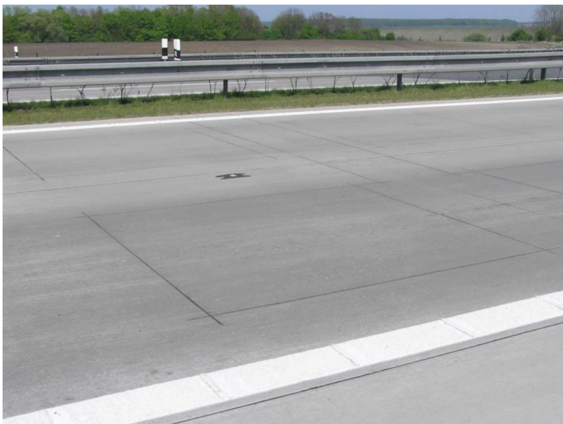
Figure 16: Rectangular induction loops for ASD3 traffic counter
