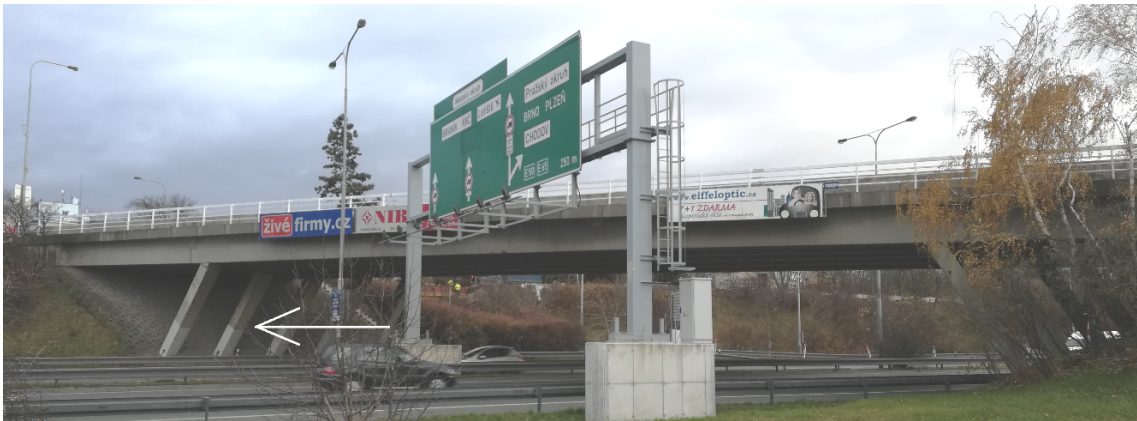
Figure 4.2: Bridge view with the analysed strut
