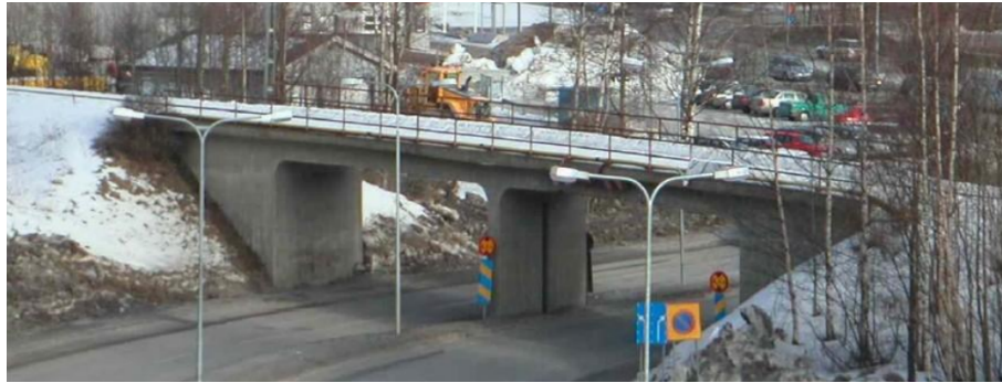
Figure 4.48: View of the bridge [44]
