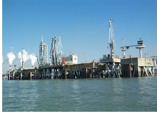
Figure 2.22: View of wharf structures [51]
