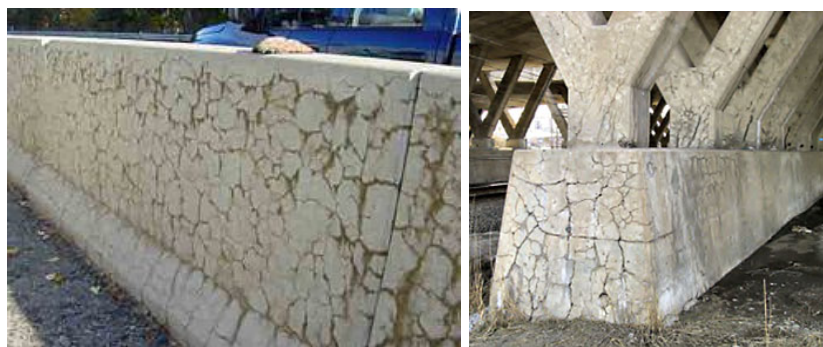
Figure 2.32: Expansion of material due to ASR reaction [120] [32]
