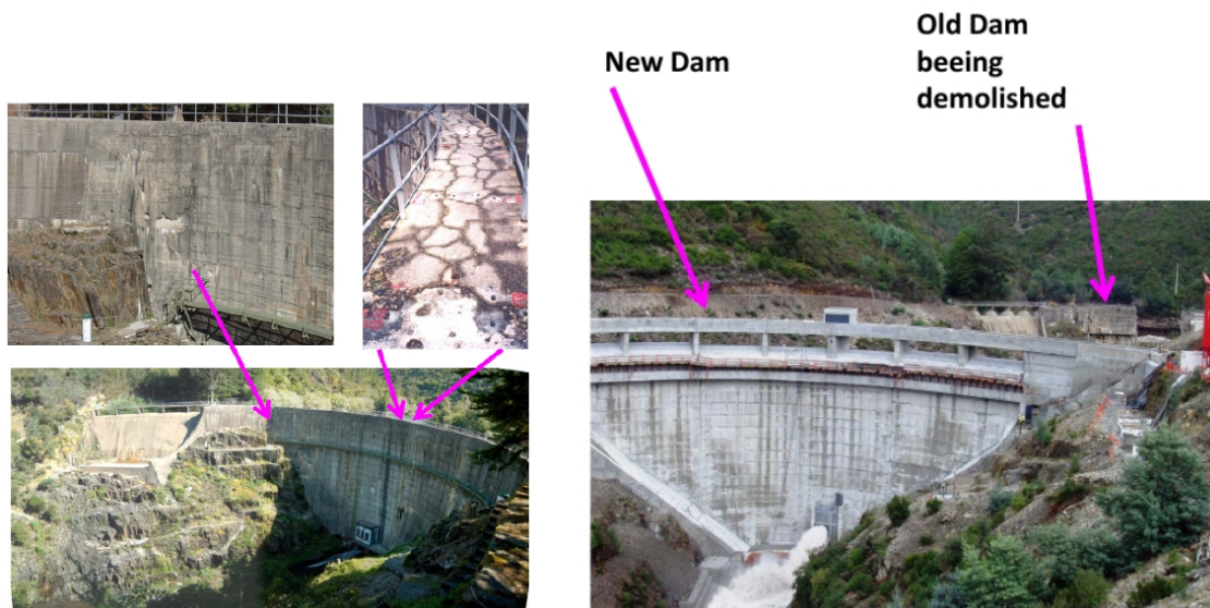
Figure 2.34: Alto Ceira dam demolished in 2012 due to excessive ASR
