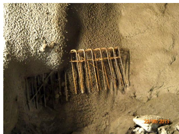
Fig. 39 Continuity bars 'kwikastrip' (left), self-prefabricated bent continuity bars (right) - installation during topheading excavation
