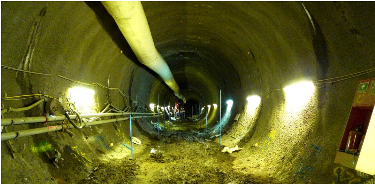
Fig. 24 In-tunnel depressurization in the pilot tunnel
