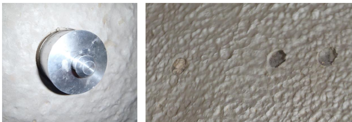
Fig. 52 Pull-out dolly (left and membrane after test (right)
