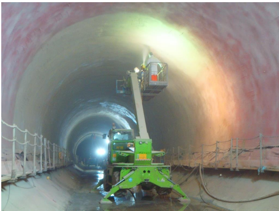
Fig. 29 Application of spray-applied waterproofing membrane in the tunnel crown
