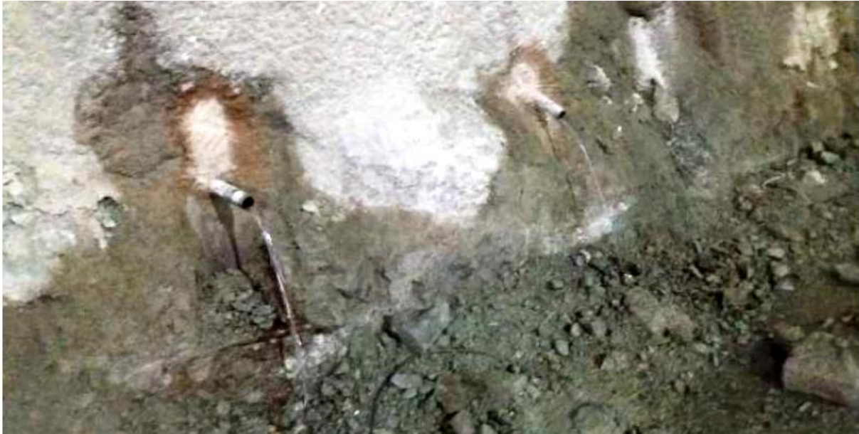
Fig. 38 Groundwater drainage intervention – drainage holes
