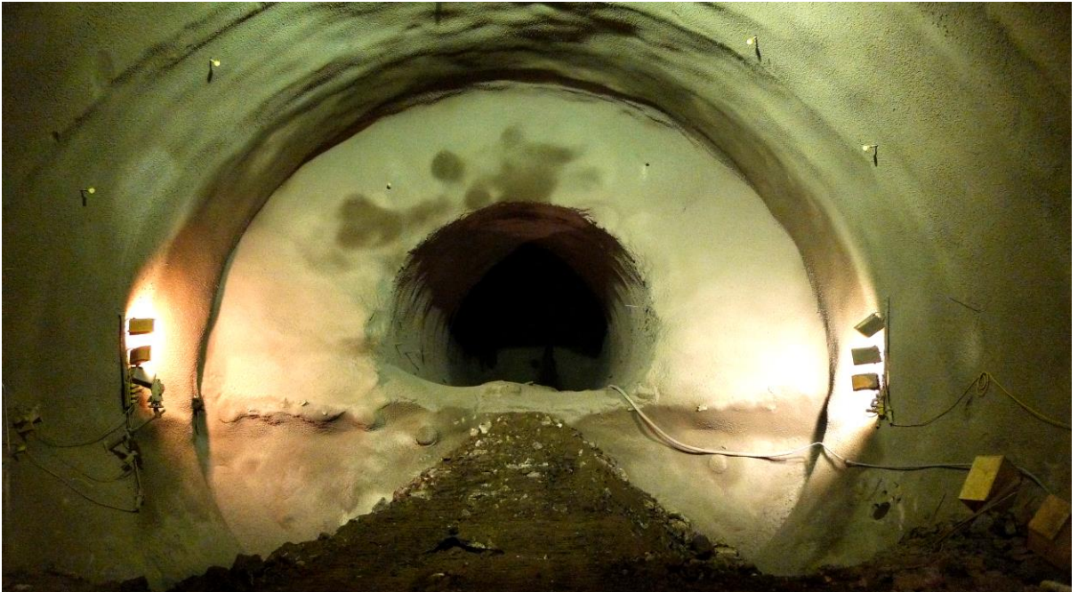
Fig. 23 Pilot tunnel excavation followed by platform tunnel enlargement
