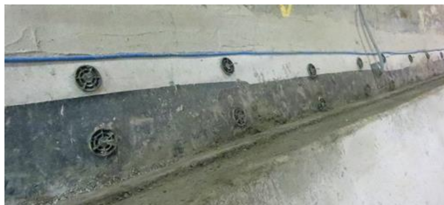
Fig. 66 Sheet and spray-applied waterproofing membrane connection detail
