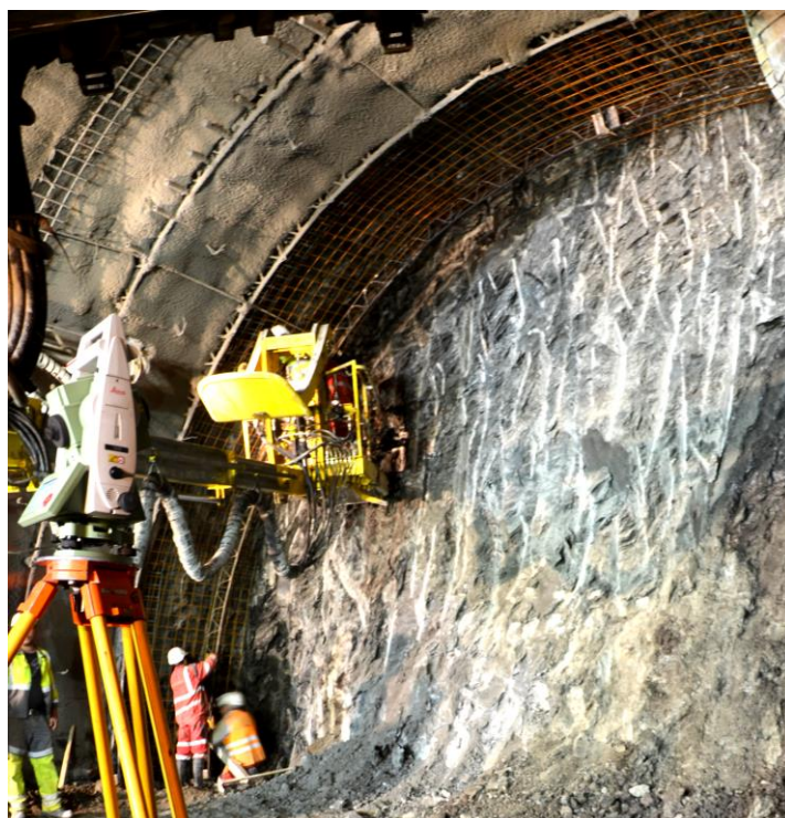
Fig. 6 NATM tunnel – installation of lattice girder and wire mesh
