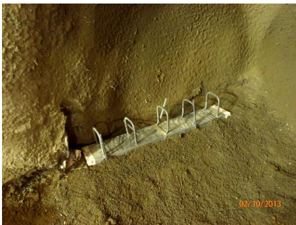
Fig. 39 Continuity bars 'kwikastrip' (left), self-prefabricated bent continuity bars (right) - installation during topheading excavation
