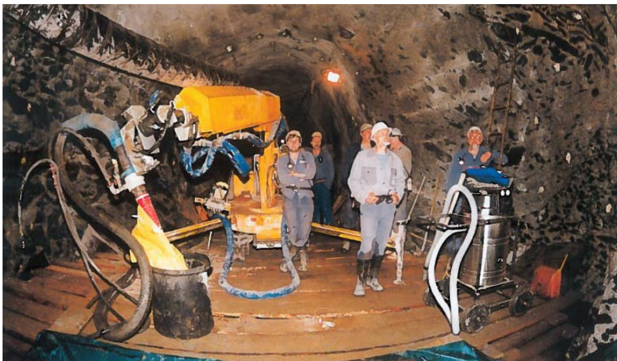
Fig. 3 Spraying robot for steel fibre reinforced concrete in 1994, [25]
