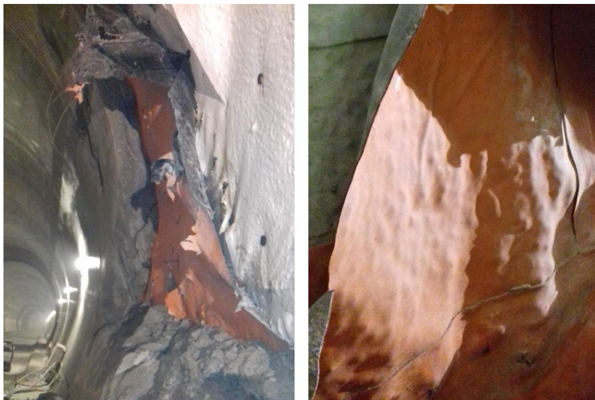
Fig. 13 Sheet waterproofing after secondary lining demolition
