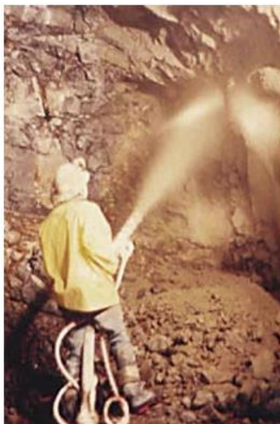
Fig. 2 Manual shotcrete application, [23]
