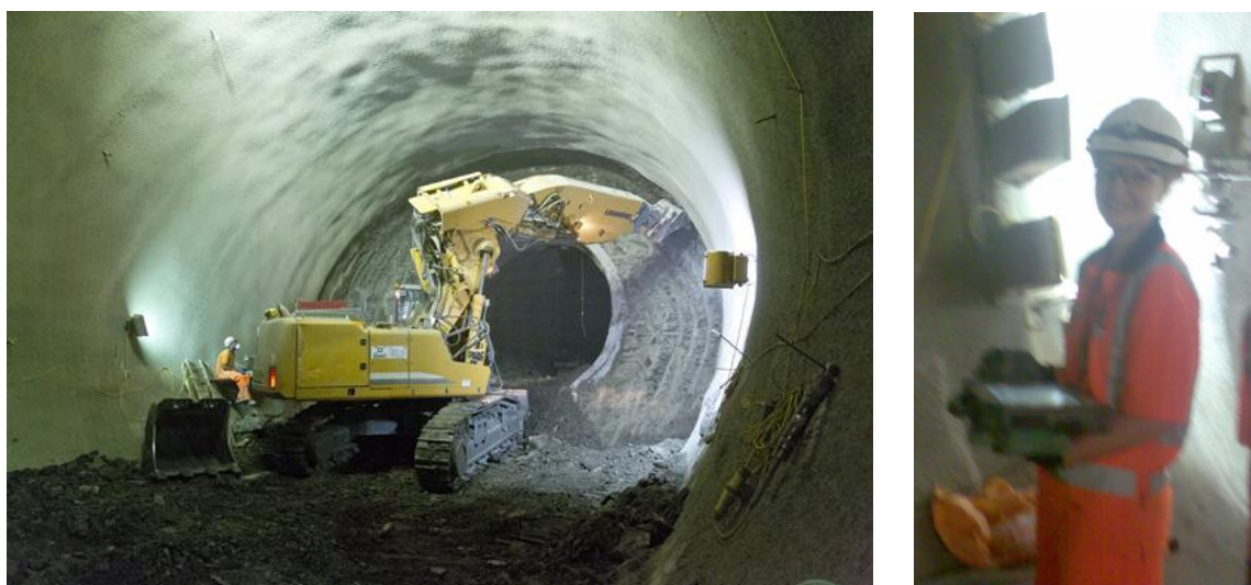
Fig. 8 LaserShell™ excavation, [35] (left), Shift Engineer with Tunnel Beamer™(right)
