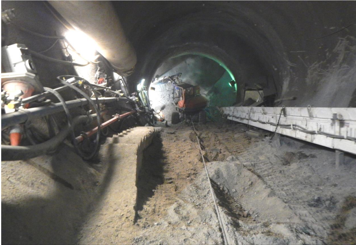
Fig. 44 Escalator tunnel with installations during construction
