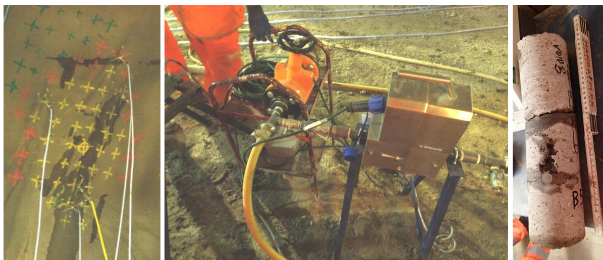
Fig. 49 Remedial works of hollow spot – injection
