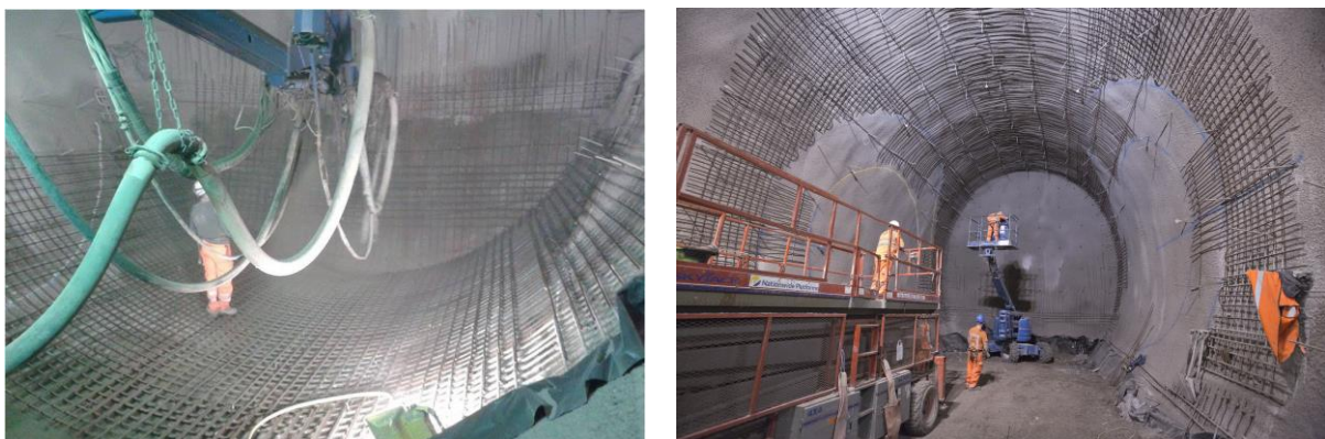
Fig. 45 Steel bar reinforced tunnel junction primary lining thickening
