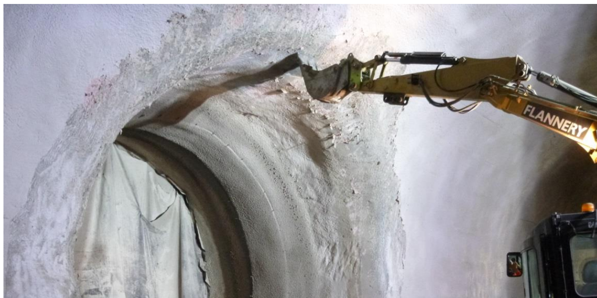
Fig. 64 Removal of overly thick membrane
