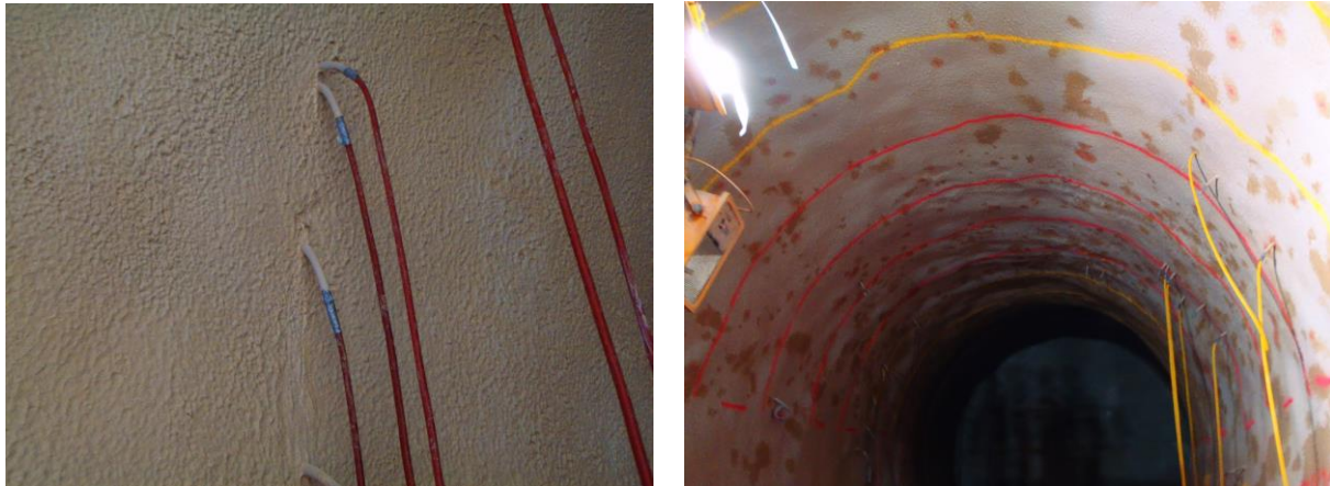
Fig. 56 Temporary spot water ingress drainage
