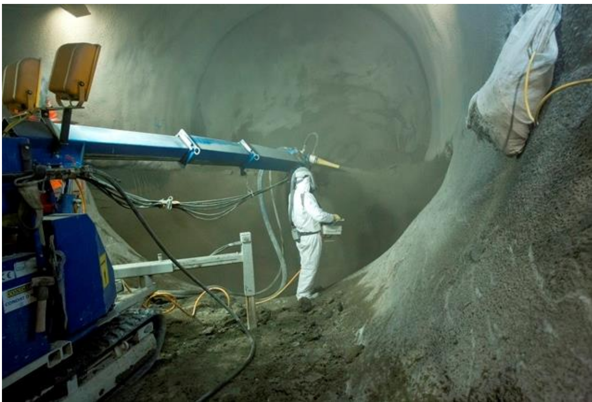
Fig. 4 Current spraying robot, [28]
