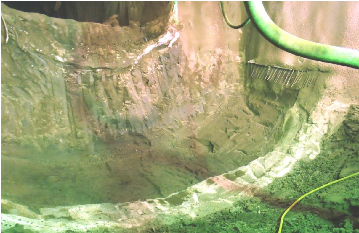
Fig. 40 Continuity bars between top-heading and invert
