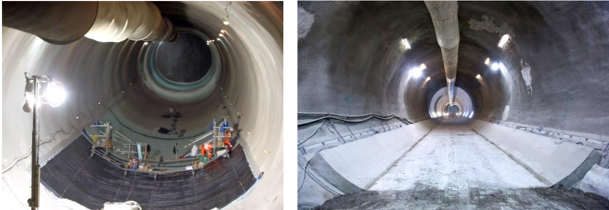
Fig. 28 Invert with sheet waterproofing membrane
