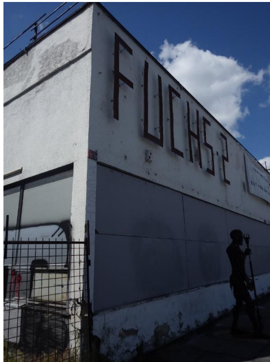
Figure 3.18: South east corner of the building with corner post
