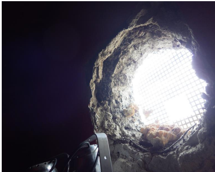
Figure 3.17: Exterior wall penetration at northeast corner of level 2NP
