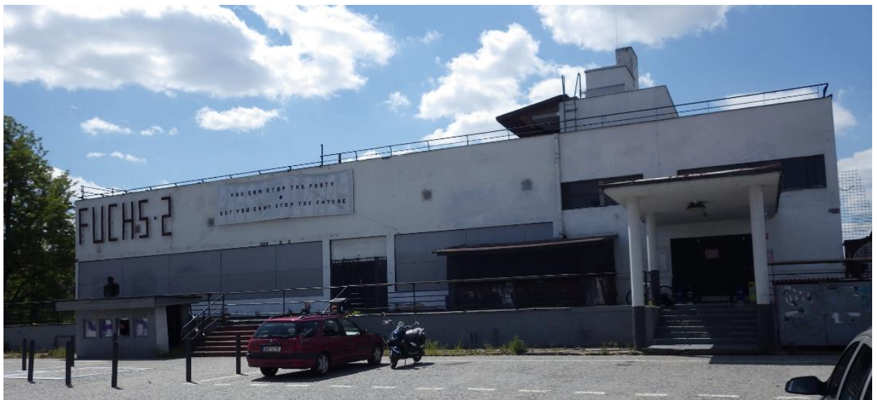
Figure 2.13: Current Exterior and Interior of Building, view from the northeast
