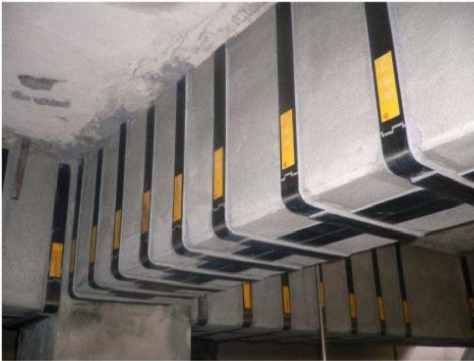
Figure 9.3: GFRP shear beam reinforcing [26]
