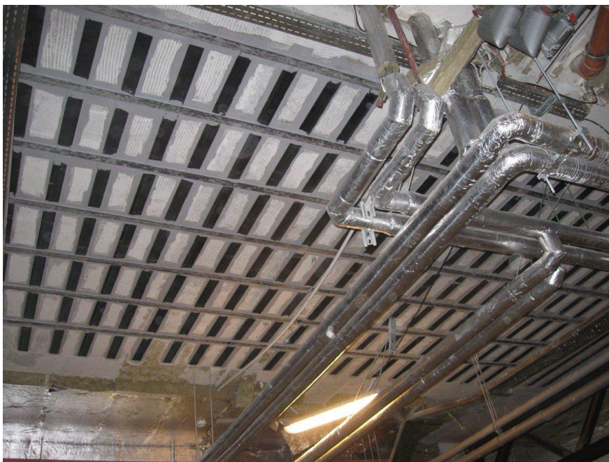
Figure 9.1: Example of CFRP slab reinforcement [25]
