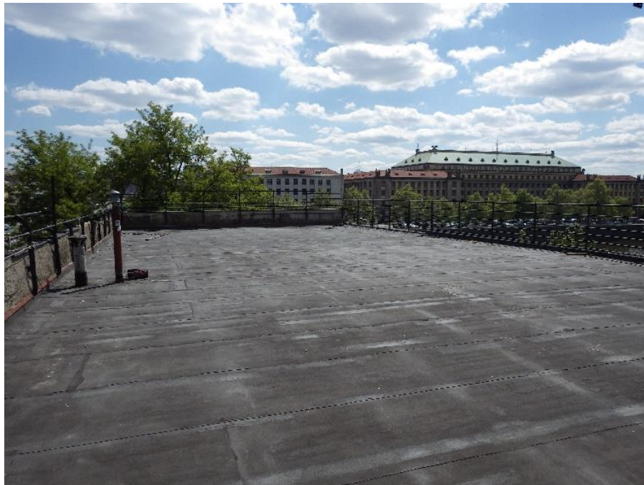
Figure 3.14: Roofing above the level 3NP slab looking south
