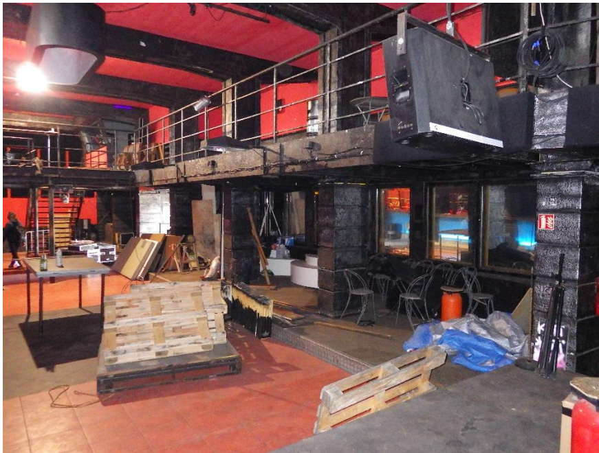
Figure 2.13: Current Interior of Building from level 1NP
