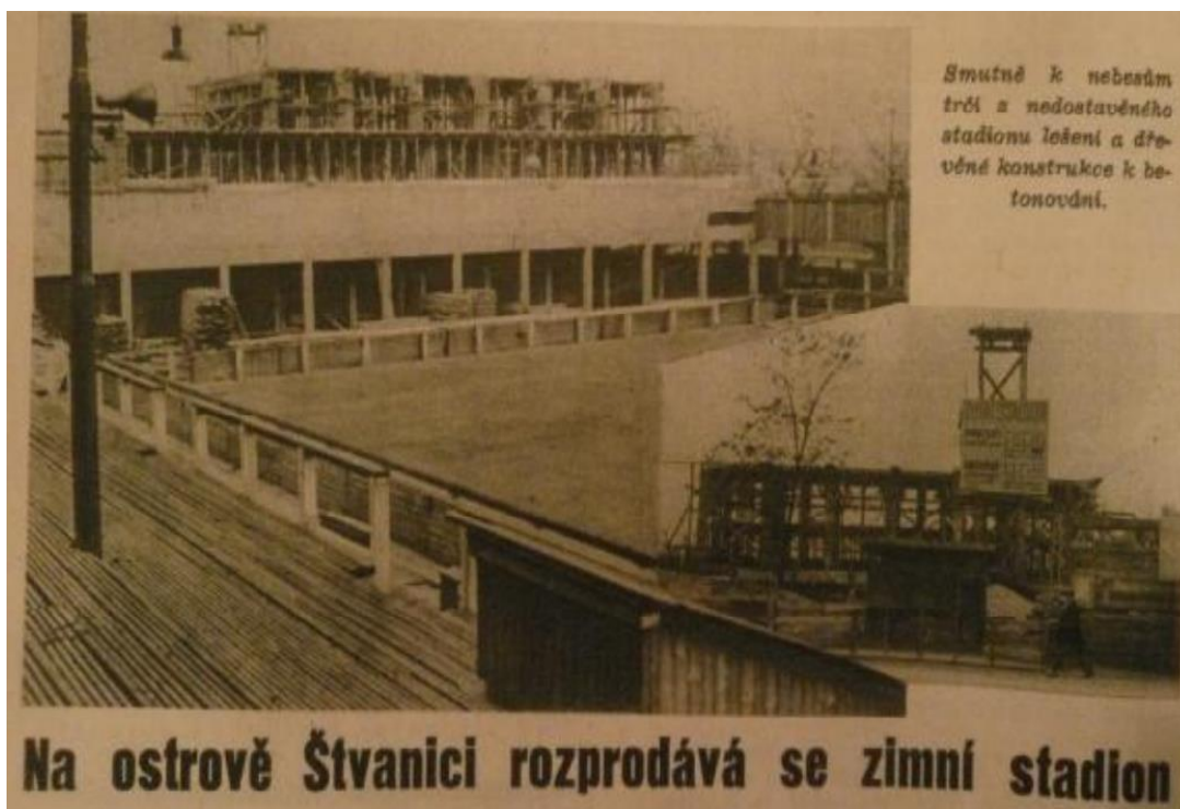
Figure 2.8: Construction Progress after Shutdown [9]
