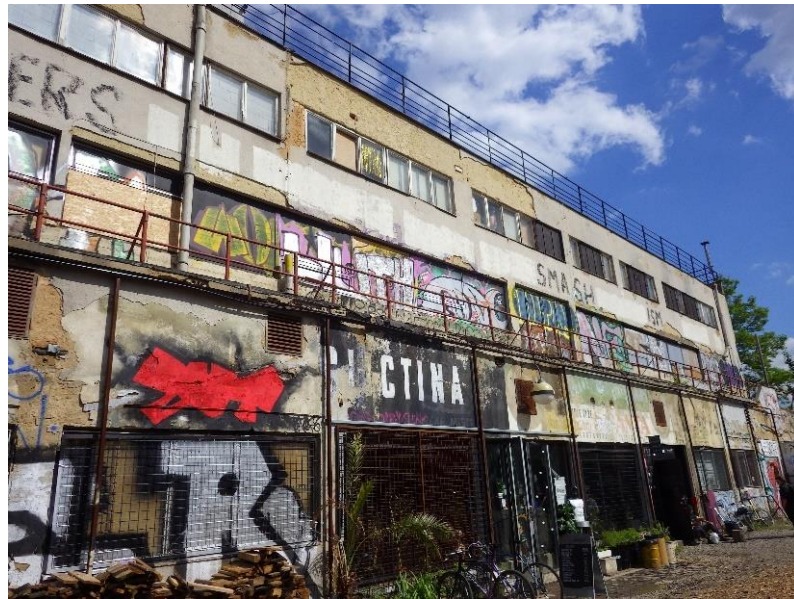
Figure 3.17: Exterior wall surface condition on western side of building
