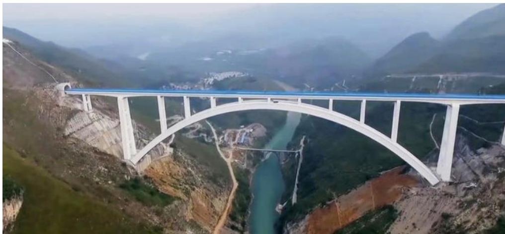
Obr. 2.25 – Pohled na most Beipanjiang Railway Bridge Qinglong [13]
