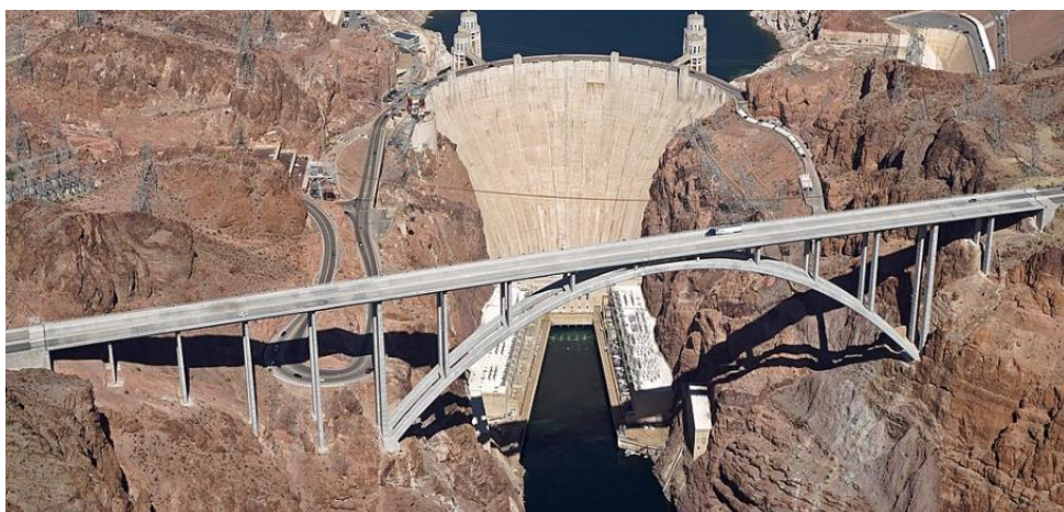
Obr. 2.22 – Pohled na most [16]
