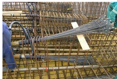
Obr. 212 Cibulová kotva [20]
