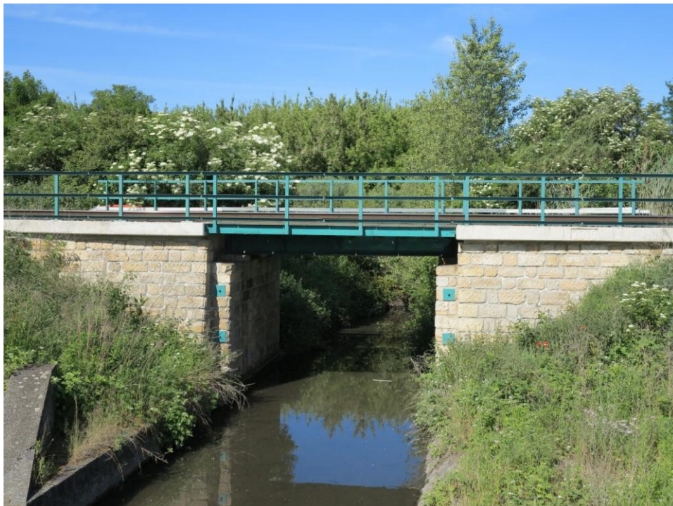
Obr. 9: Most, evid. km 20,198
