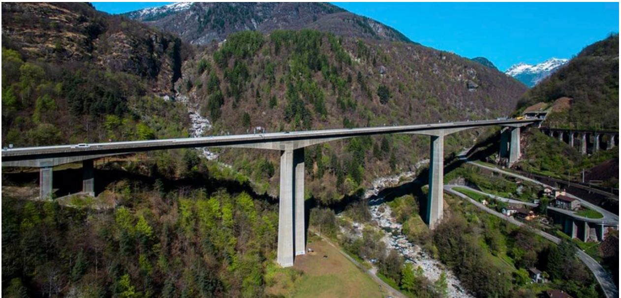
Obrázek 5.6: Biaschina viaduct, SUI [22].
