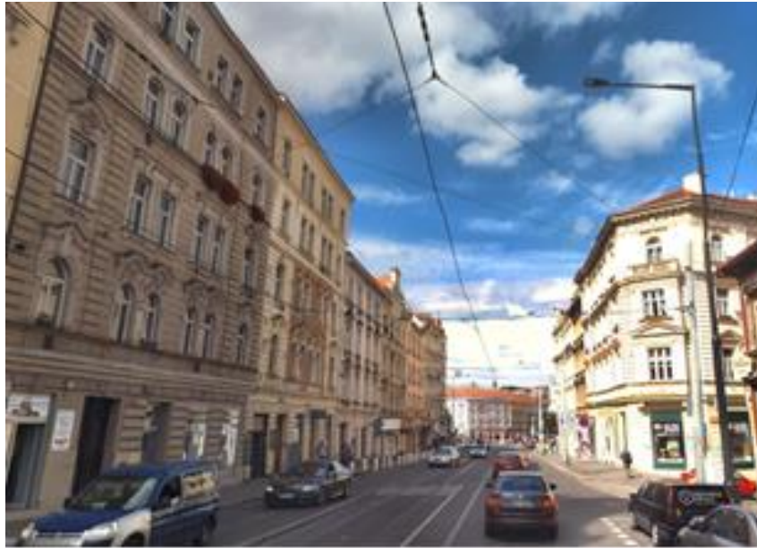
Figure 18. Nuselská street in Prague with LED in the front and HPS in the back
