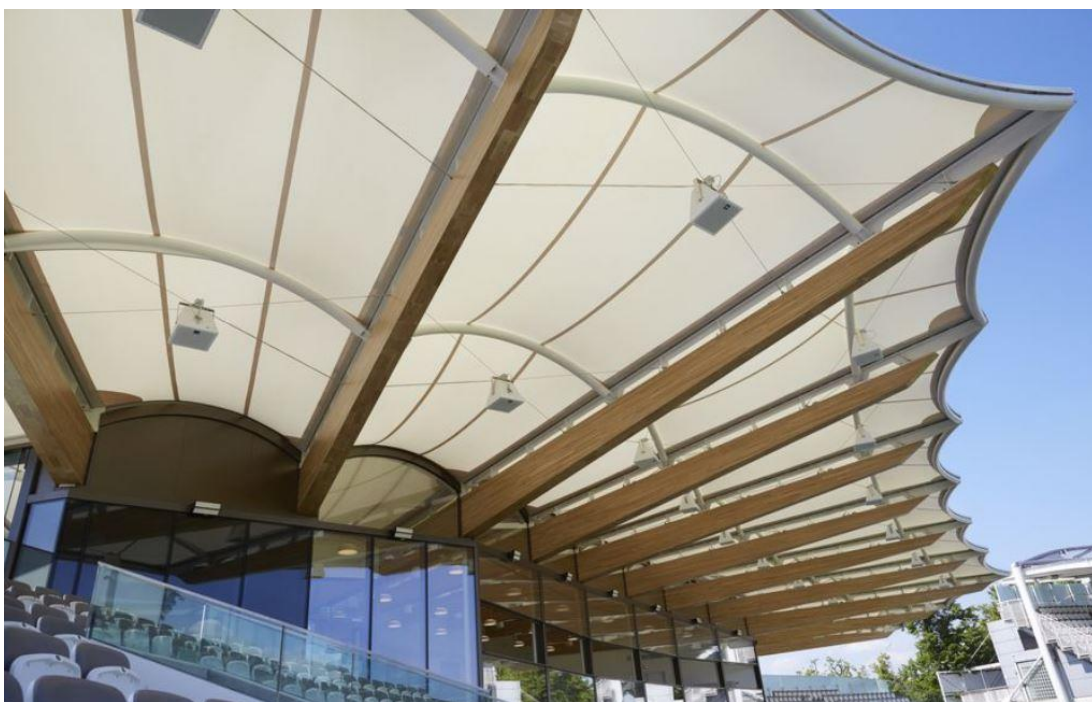
Obrázek 47 – Lord's Cricket Ground – pohled na vazníky [30]
