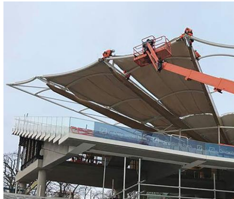
Obrázek 51 – Lord's Cricket Ground – instalace membrány [33]
