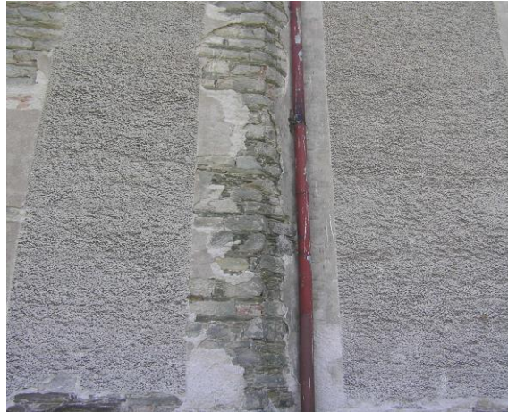
Picture 34: Discoloration of the external wall and missing render (St. Barbara's Church)
