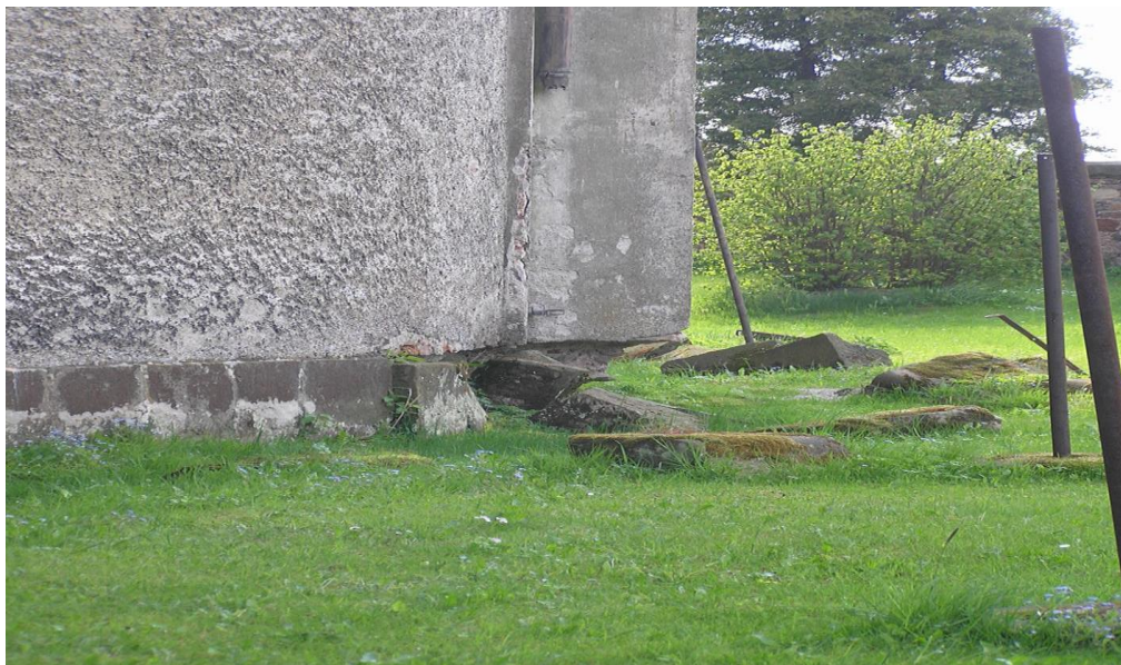
Picture 31: Cracks, render loss and erosion of the stones (St. Anna's Church)
