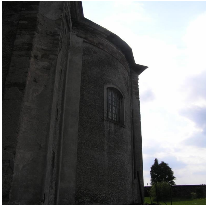
Picture 31: Cracks, render loss and erosion of the stones (St. Anna's Church)
