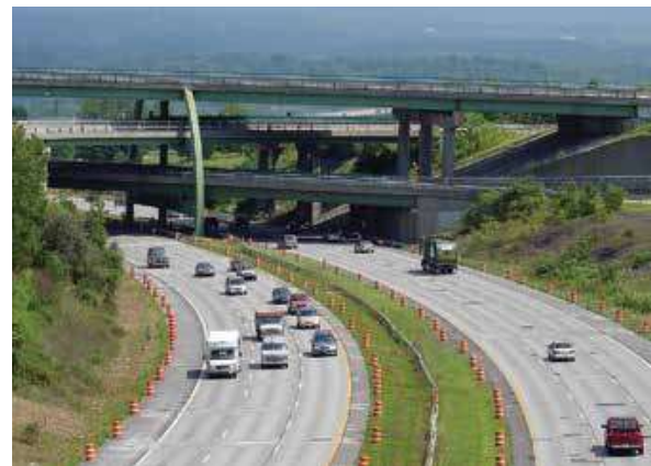
Figure 4: JPrCP installed intermittently in horizontal curves.
