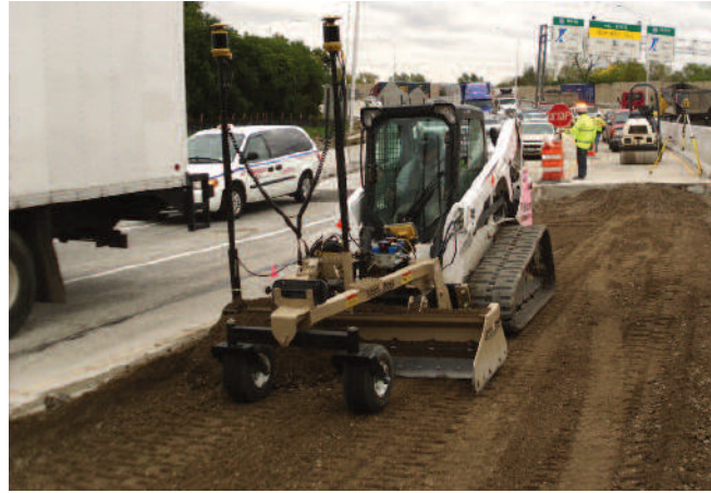
(left) laser-controlled skid steer for large scale supergrading
