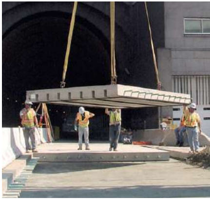
Fig. 10 : Fort Miller Super Slab System [22] Fig. 11 : Fort Miller Super Slab - Joint detail [22]
