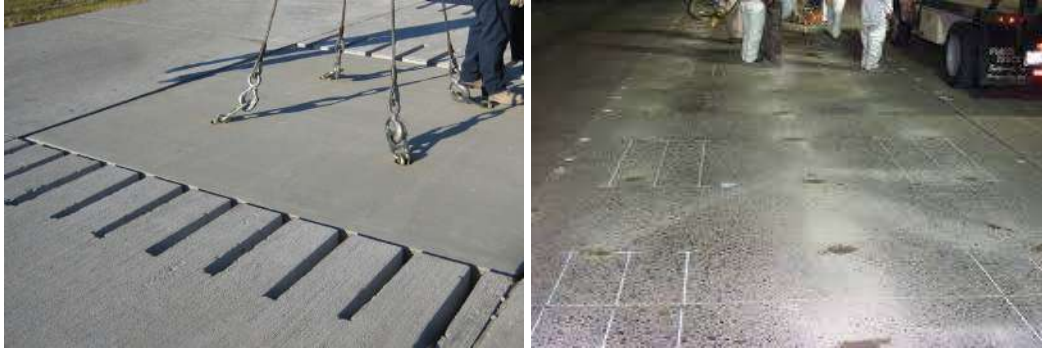
Fig. 12 : URETEK Method System [GooglePhotos] Fig. 13 : URETEK Stitch-In-Time System [GooglePhotos]
