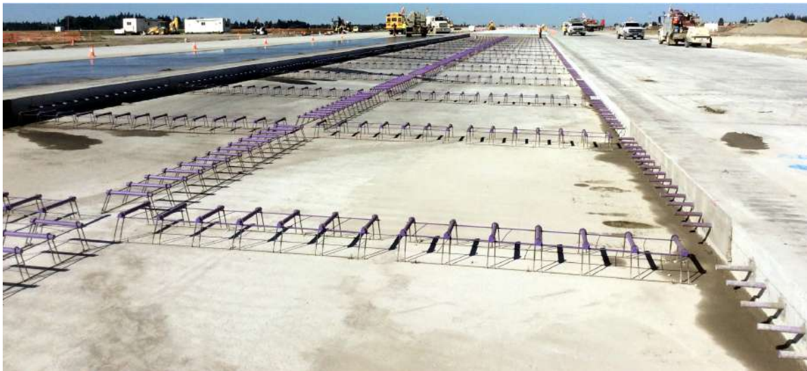
Fig. 5 : JRCP - Jointed Reinforced Concrete Pavement [GooglePhotos]
