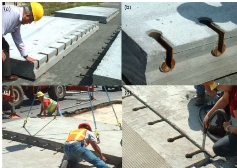
Fig. 14 : Kwik Slab System - (a) female-type and male-type components of interlocking system; (b) steel connector sockets; (c) panel installation; (d) injection of high-strength grout. [20]
