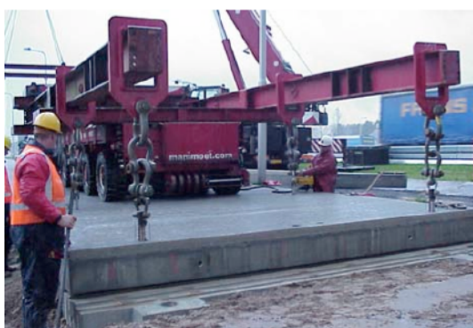
Fig. 16 : Modie Slab System [19]
