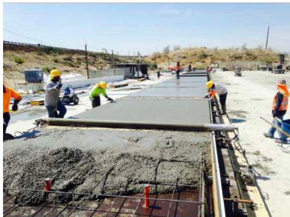
Fig. 9 : Pre-cast panels fabrication [22]
