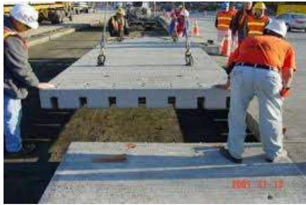
Fig. 10 : Fort Miller Super Slab System [22] Fig. 11 : Fort Miller Super Slab - Joint detail [22]
