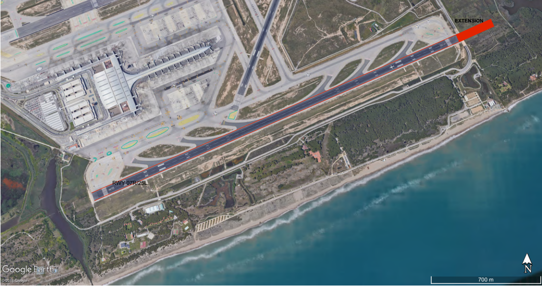
Fig. 27 : View of runway RWY 07R/25L surface with represented extension (GoogleEarth)
