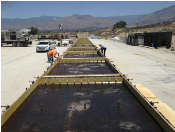
Fig. 8 : Pre-cast panels formwork [22]
