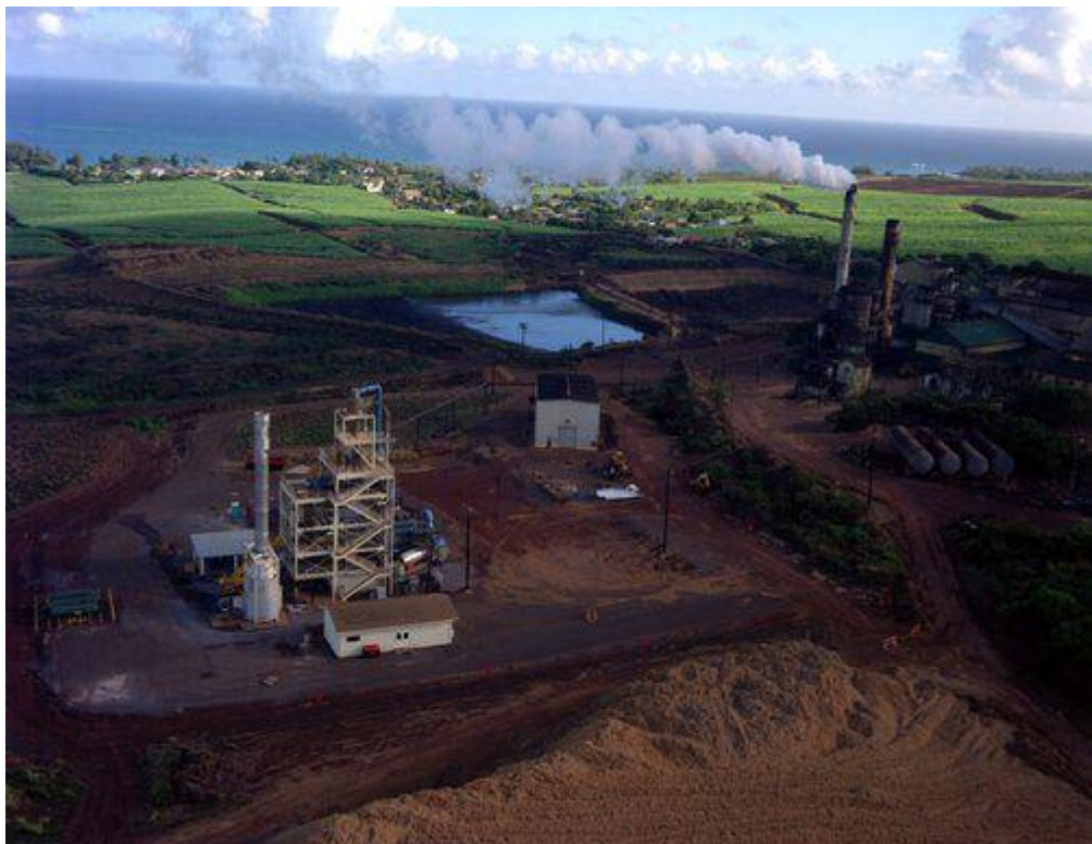
Fig. 22 Gasification plant in Maui, Hawaii [24]
