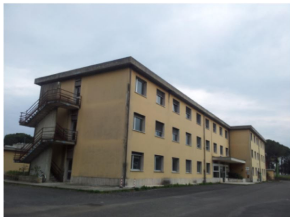
Figure 4.a: Front view of ENEA building
