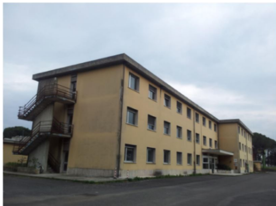
Figure 4.a: Front view of ENEA building
