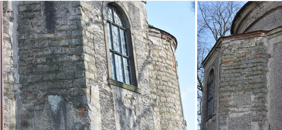
Figure 3.5. Uncovered wall facade
