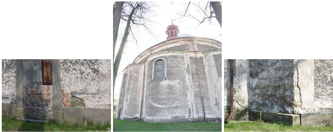
Figure 4.8. Efflorescence
