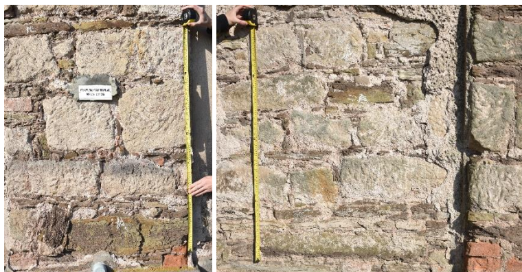
Figure 5.1. Two different parts of the enclosure walls that were tested
