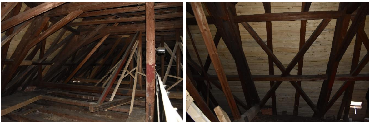
Figure 3.3. Roof truss in the Church
