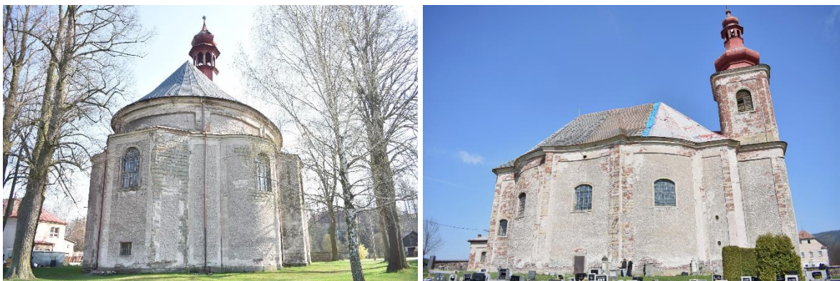
Figure 4.1. Facades of St Barbara Church (left) and St Anna Church (right)
