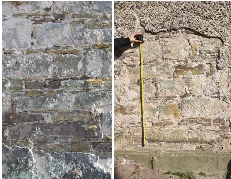
Figure 4.5. Material Loss
