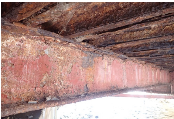
Figures 12 and 13. Bridge Condition: Corrosion of the Bottom of the Deck (left); Light Corrosion on the Section Over the Deck (right).
