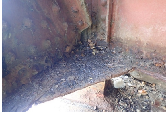
Figures 10 and 11. Bridge Condition: Accumulation of Debris (left); Gusset Plate Corrosion (right).
