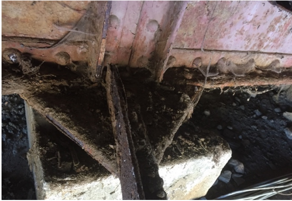
Figures 10 and 11. Bridge Condition: Accumulation of Debris (left); Gusset Plate Corrosion (right).
