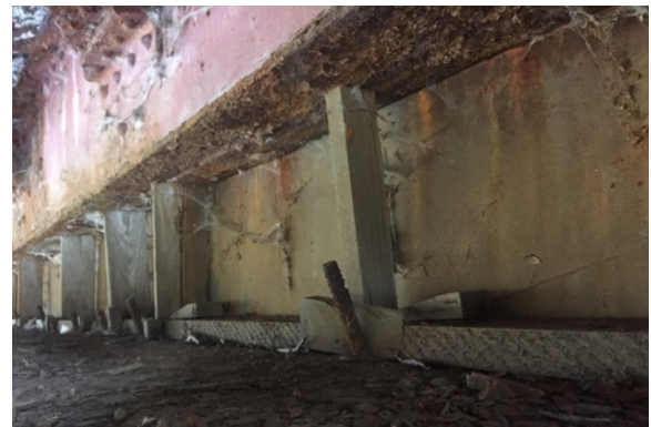
Figures 14 and 15. Previous Repairs: Asphalt Layer (left); Temporary Wooden Supports (right).
