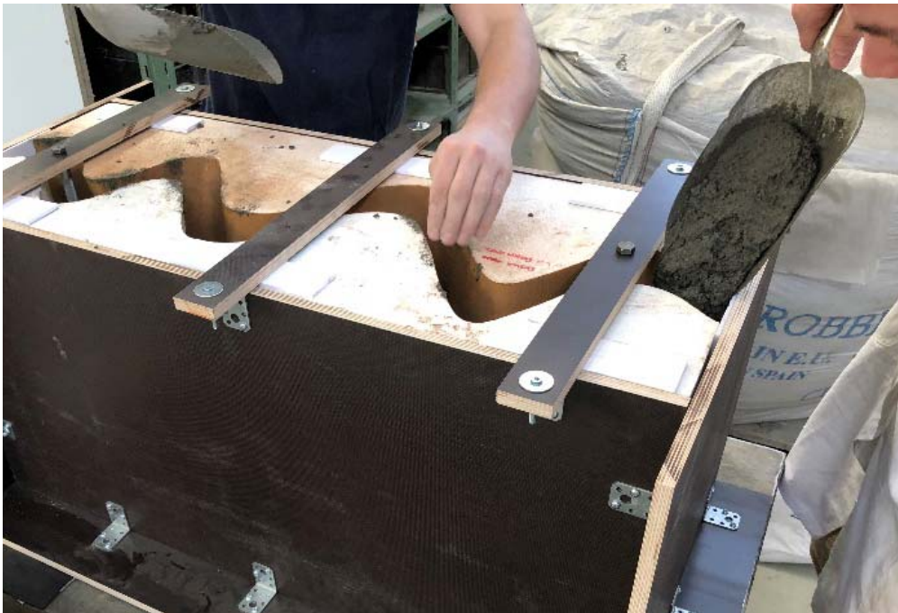
Fig.56 Pouring. Source: author
