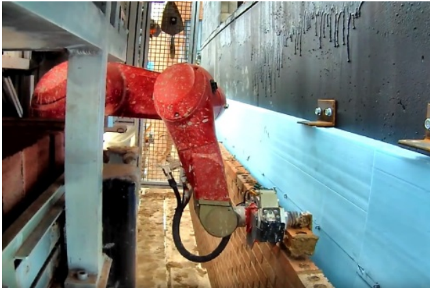
Fig.11 Bricklaying by „SAM“. Source: [20]
