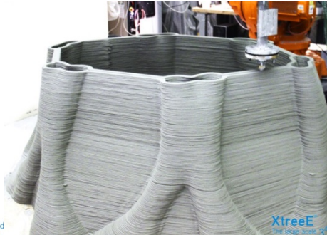
Fig.16 Manufacturing of post.
