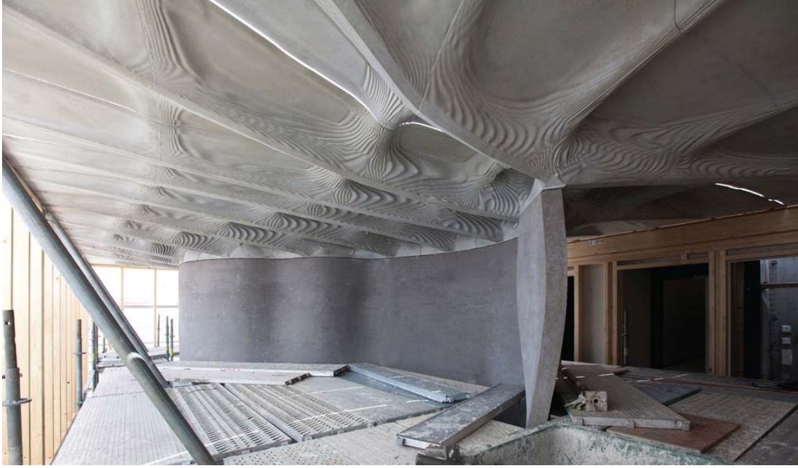
Fig.28 Assembled slab. Photo: [8]
