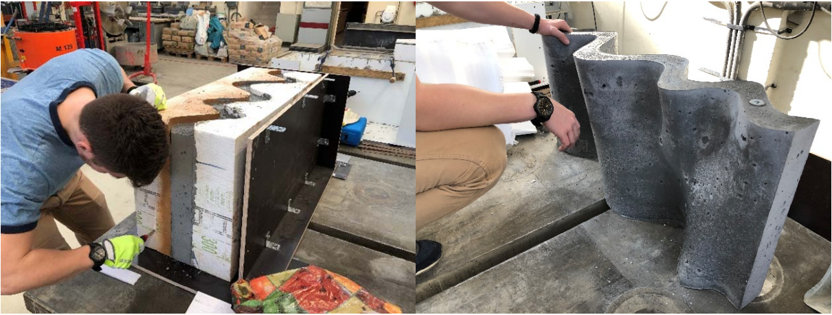
Fig.57 Removing the formwork. Source: author
