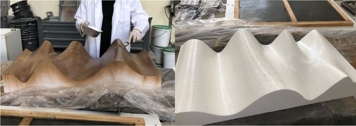
Fig.53 Coating the EPS formwork surface. Source: author
