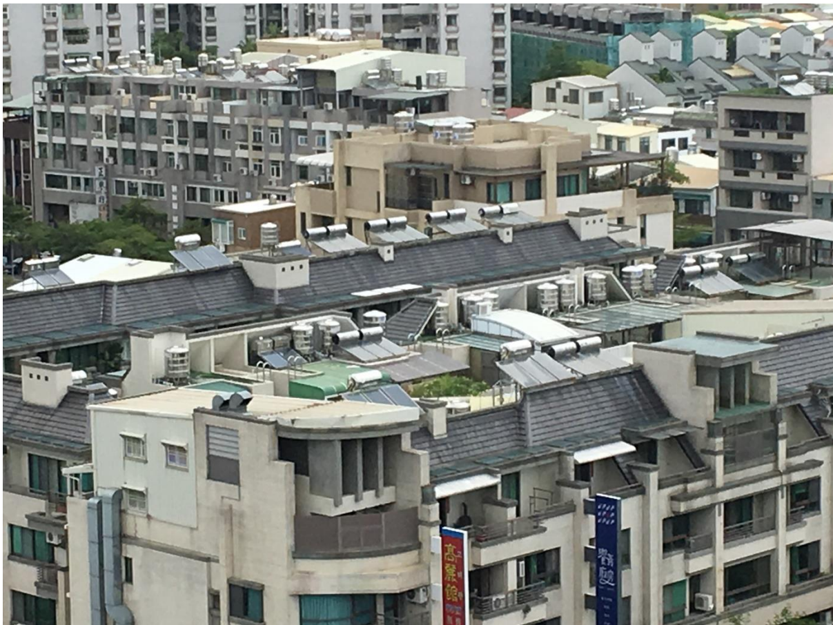
Pic. 22: Rooftop water storage – steel tanks, Tainan, Taiwan
