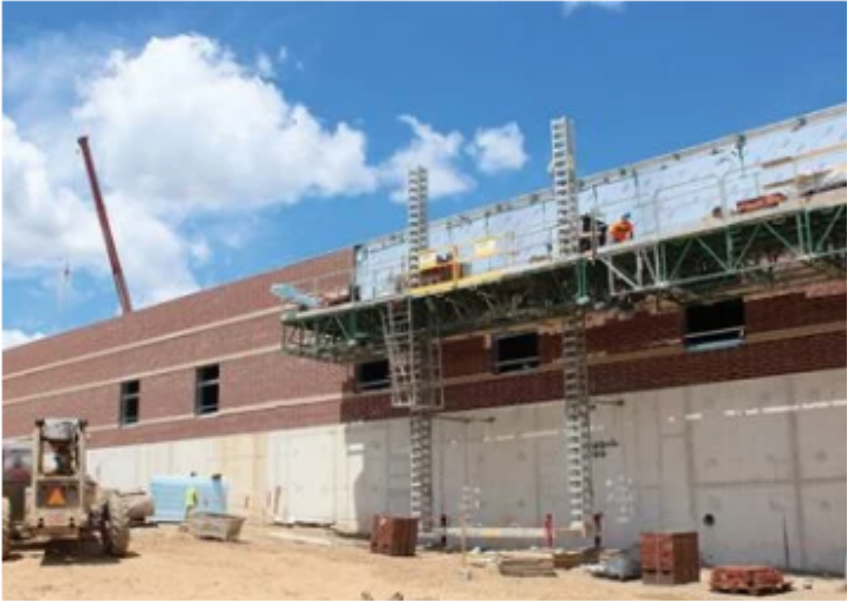
Fig. 49 SAM100 utilized for construction of a building. 169
