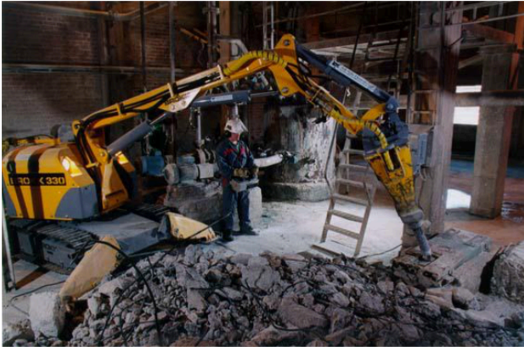
Fig. 19 Demolition process with the help of a robot. 99
