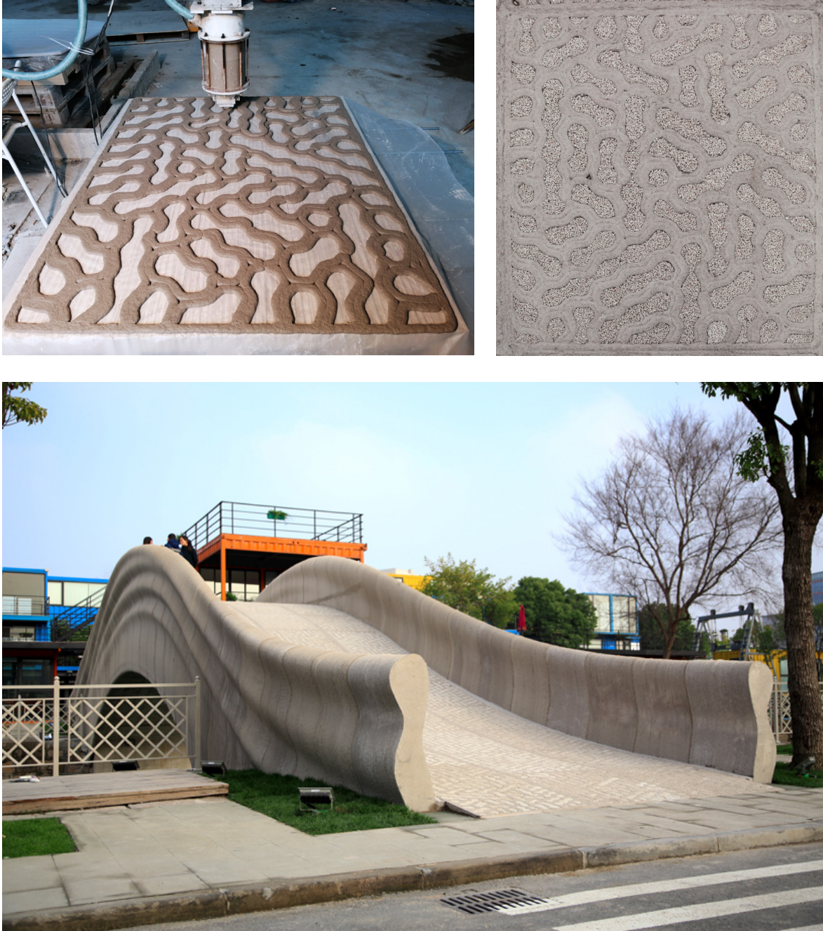
Fig. 38b The process of building the bridge pavement. 142
