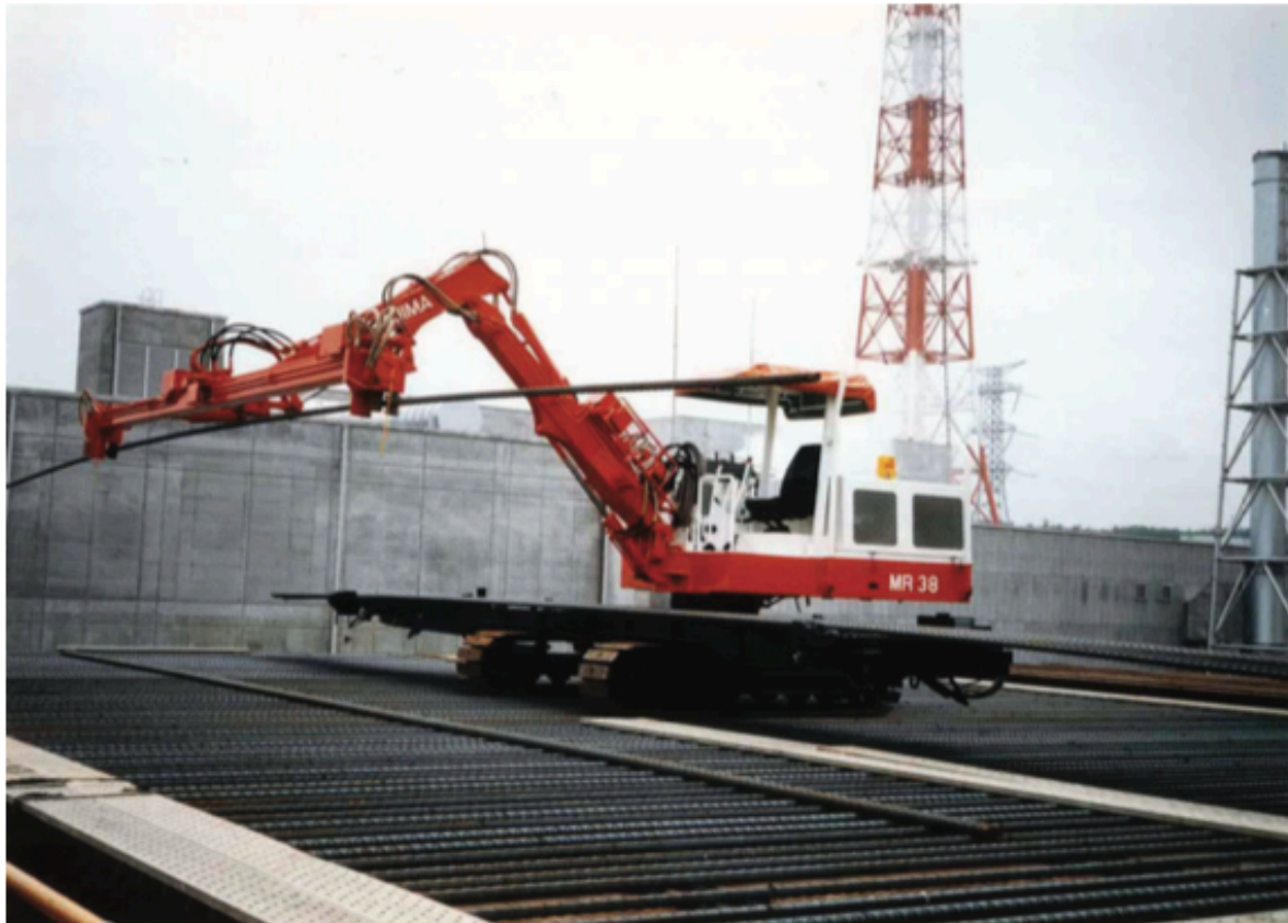
Fig. 39 Reinforcement positioning robot. 144
