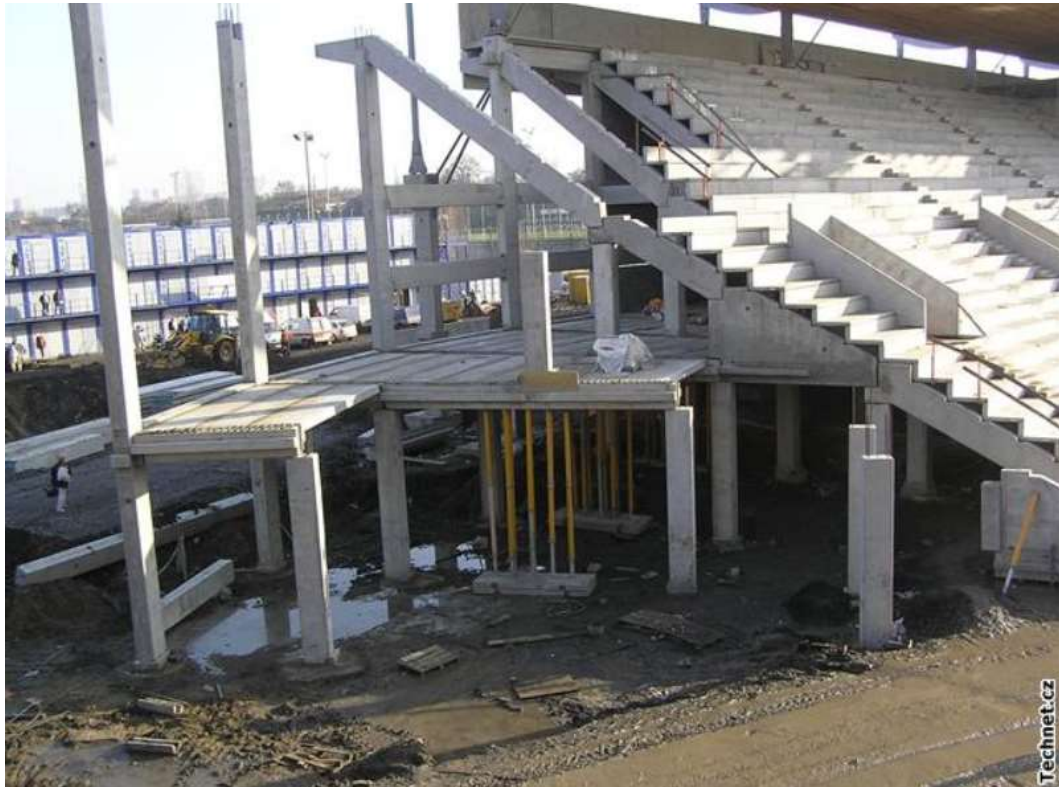
Obr. 3.3-6 – Sinobo Stadium, Praha, ČR [38]
