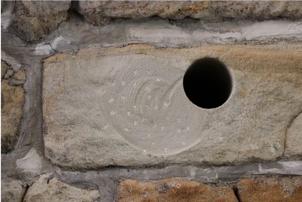
Fig. 12 Grinded rock surface prepared for measurement right next to borehole. Visible dots are caused by hammer impacts. (picture: M. Jonáš)
