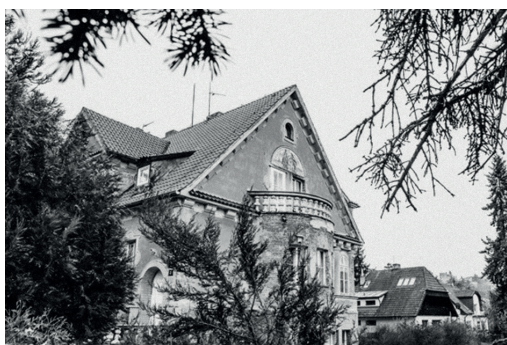
Unique rondocubist villa. The adaptation of the older building from the 19th century was carried out in the years 1921-1922 according to Pavel Janák's project in cooperation with the artist František Kysela.
