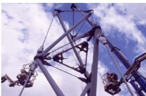
Obr. 2.3c Warnow Tower – montáž, temporary stressing frame [4]
