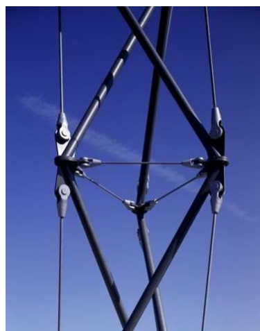
Obr. 2.3b Warnow Tower – detail [105]
