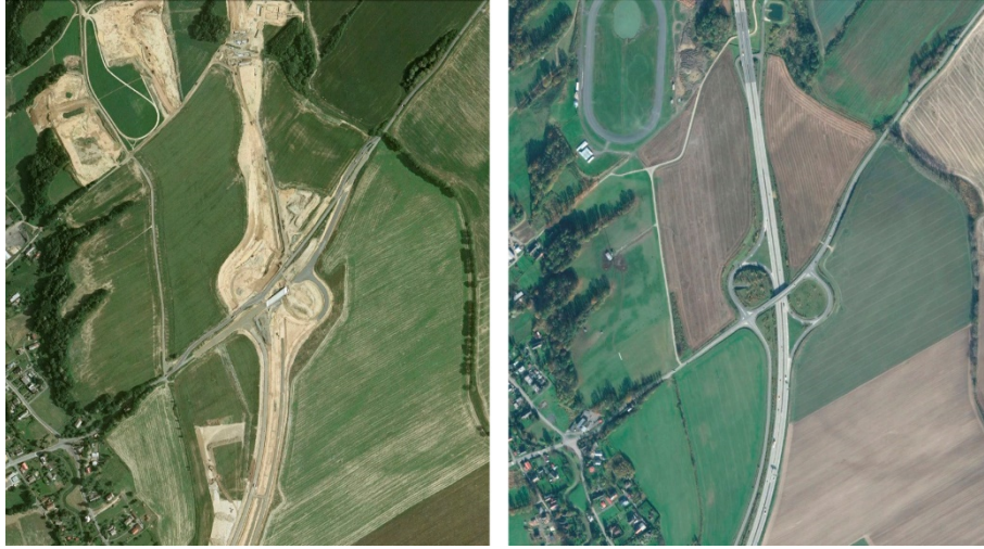
Figure 59. Construction of the D1 near Ostrava in 2006 (left). The same section in operation in 2018 (right). (Source: Google Earth ©, accessed December 10, 2018).
