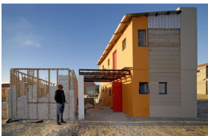
Obrázek 5: 10x10 Housing Initiative, Sandbag houses (JAR)
