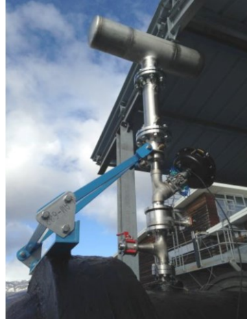
Figure 3 Degassing system for Thermosiphon condenser
