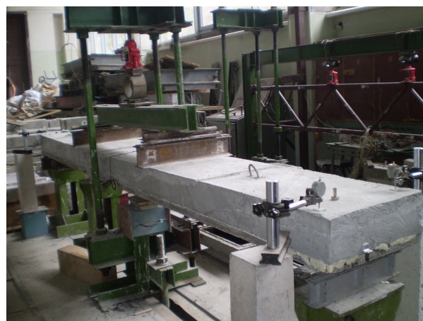
FIGURE 5. The look of experimental facility during study of sandwich reinforced concrete-foamed concrete floor slabs.
