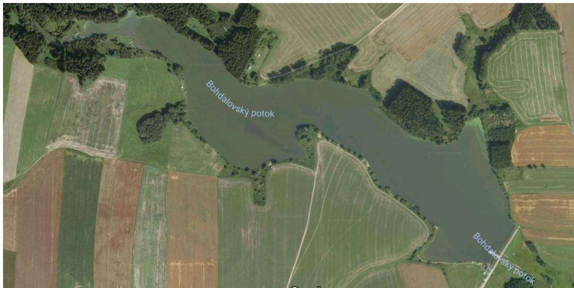
Figure 34 - Water reservoir Ostrov nad Oslavou [31]
