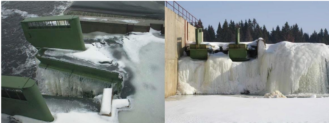
Figure 21 - Fuse gates in winter conditions (Khorobrovskaya Dam) [26]
