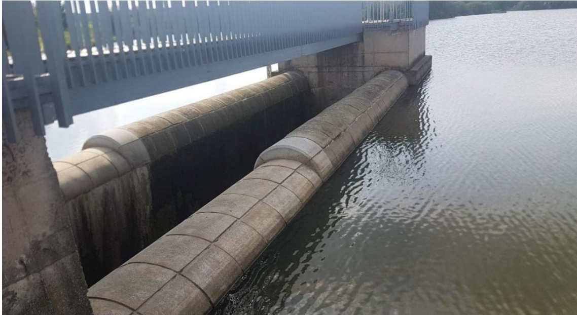
Figure 31 - Curved spillway crests [30]
