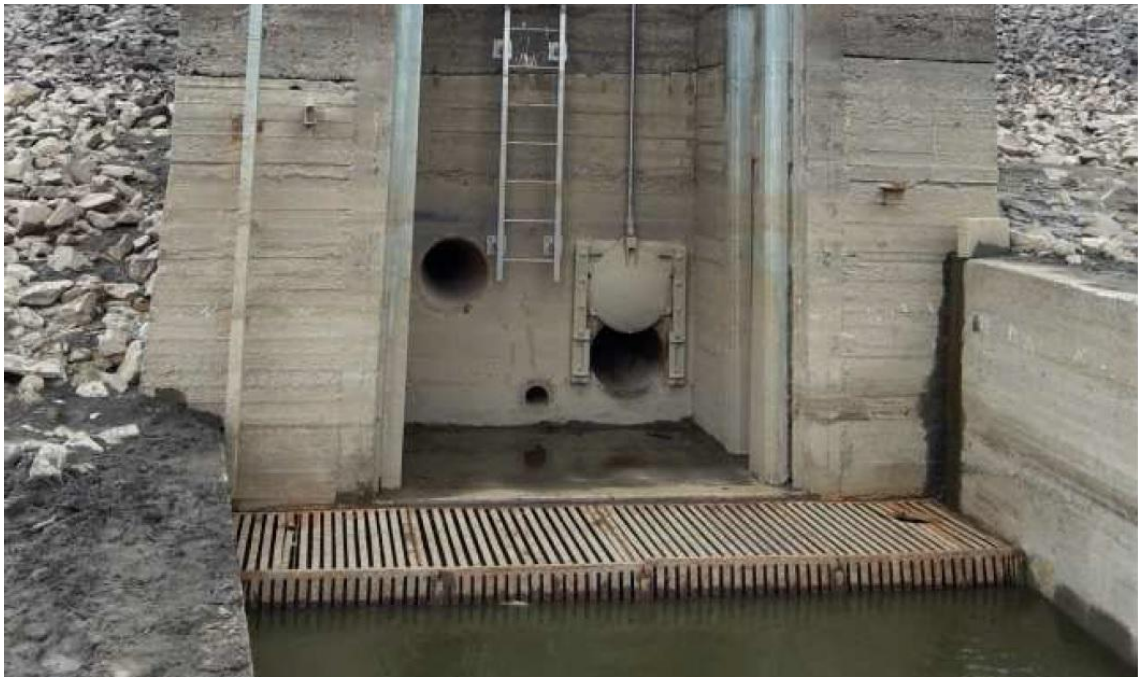
Figure 30 - Bottom outlets and the upstream side of the operation shaft [29]
