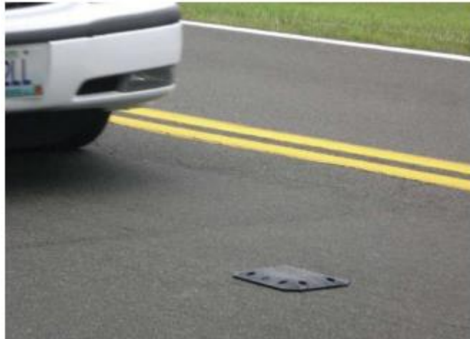
Figure 6.: Magnetic detector attachment on pavement [9]
