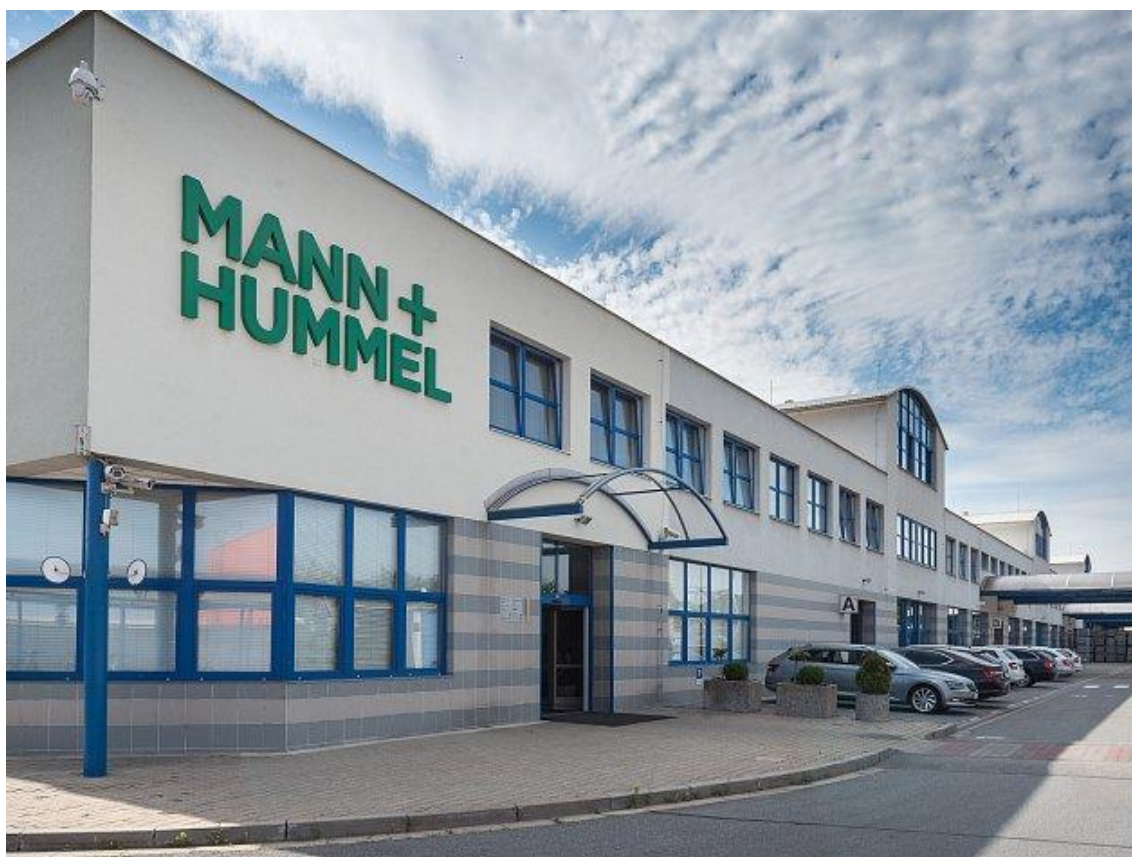
Obr. 1: Budova firmy Mann+Hummel [2]
