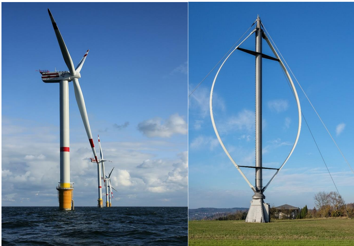
a) Horizontal-axis wind turbine
