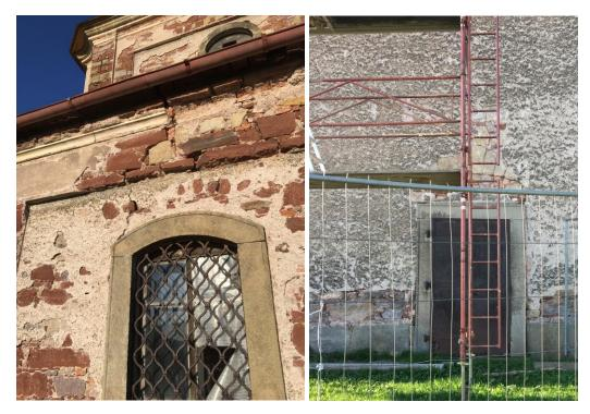
Figure 3.5 - Cracks on the exterior of the church. Sacristy (Left) Main Nave South side (Right)
