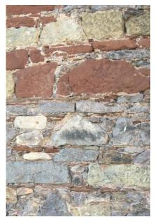
Figure 7.5 - Outer masonry wall showing missing mortar at some locations
