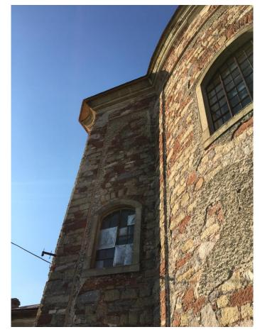
Figure 4.1 - Enclosure wall masonry from the exterior shows non-uniform combination of stones building up the outer layer
