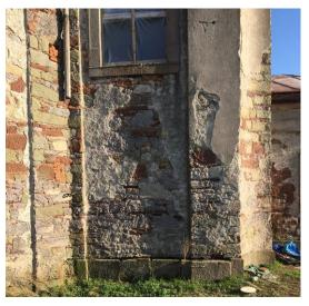
Figure 3.7 - Detachment as scaling on plasters
