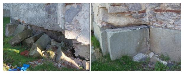
Figure 3.6 - Deformation of Northside (Left) Southside (Right)
