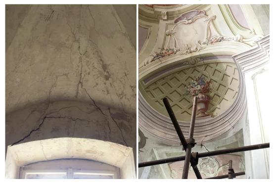
Figure 3.4 - Cracks on the Interior of the Church. Sacristy (Left) Main Nave (Right)
