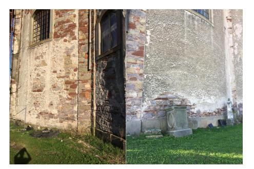
Figure 7.2 - non-performing rain water downspout (Left) damage in walls due to ground water in walls (Right)
