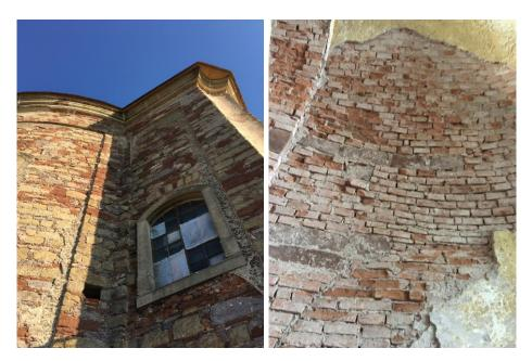
Figure 3.9 - Plaster loss at the exterior (Left) and Interior (Right)
