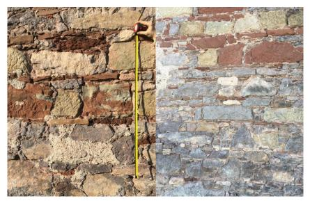
Figure 3.8 - Erosion of stones at the exterior side
