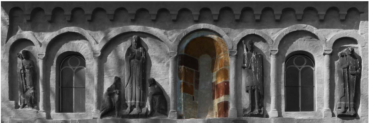
Figure 1.1.1. Remains of the original colored plaster.
