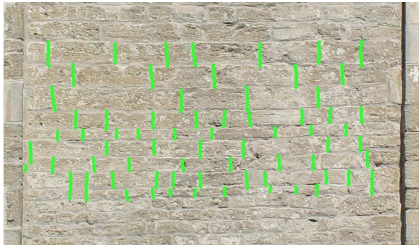
Figure 4.2.1.8. Vertical joints analysis.
