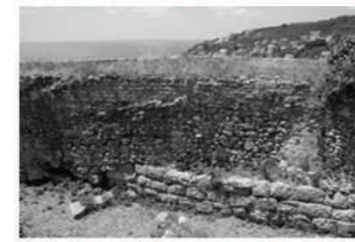
Illyrian wall BC built with large stone blocks in dry technique
