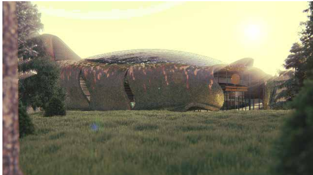
EXTERNAL view looking at the weathered and foliage covered facade
