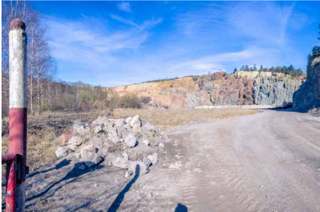
VIEW FROM THE ROAD View looking up from the base level at the gate to the site
