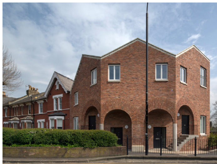
Stephen Taylor Architects
