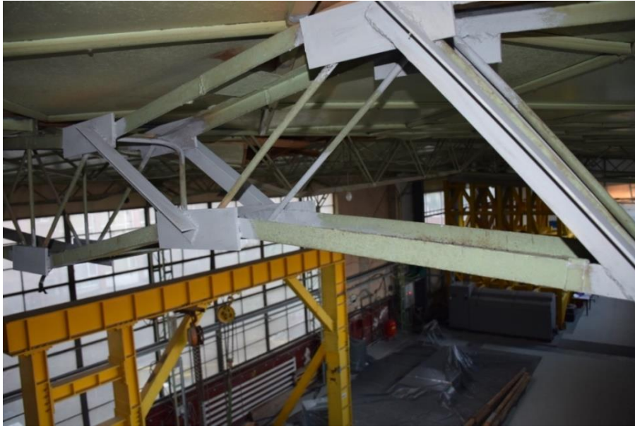
Figure 4.2 The girder from the frame in axis 4 after the partial rehabilitation
