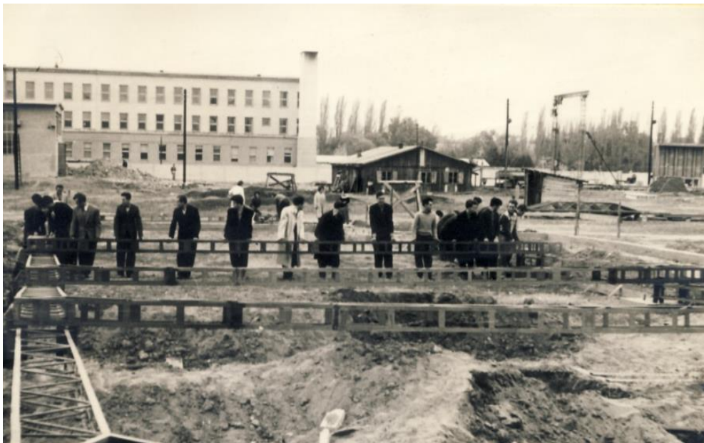
Figure 2.1 Erection of the steel structure [5]
