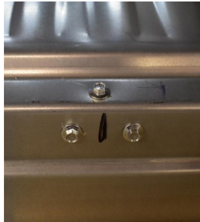
Figure 3.7. Overlap fixing
