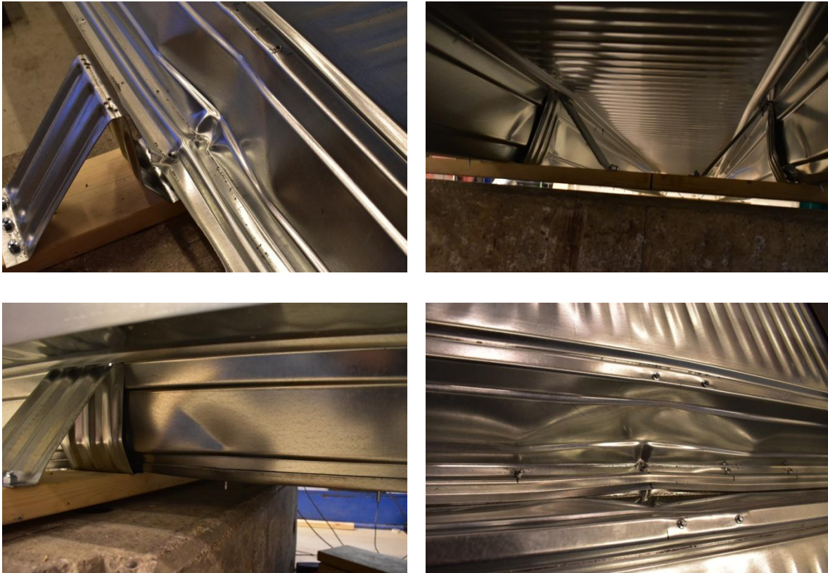
Figure 3.24. Failure of 1.50mm Test Set-up 1
